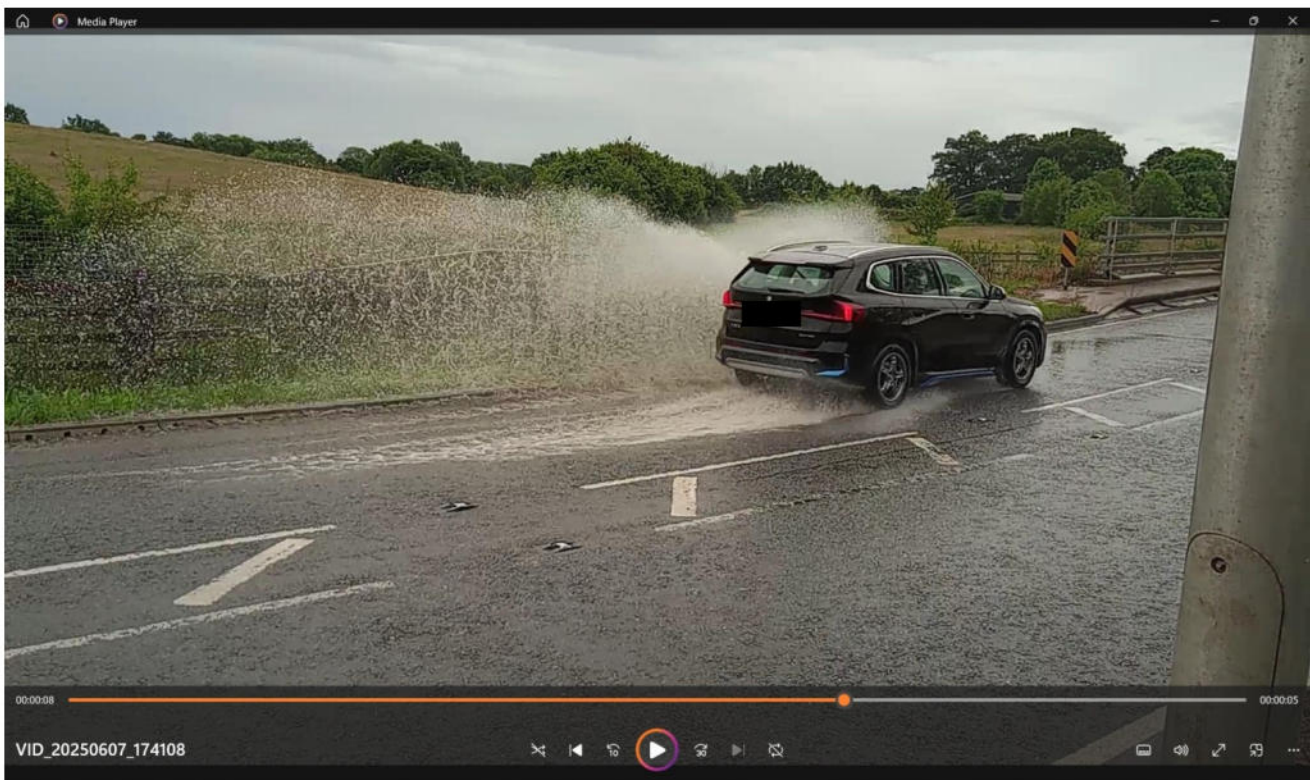
Image 12 - standing water on the highway, east of the bridge:
