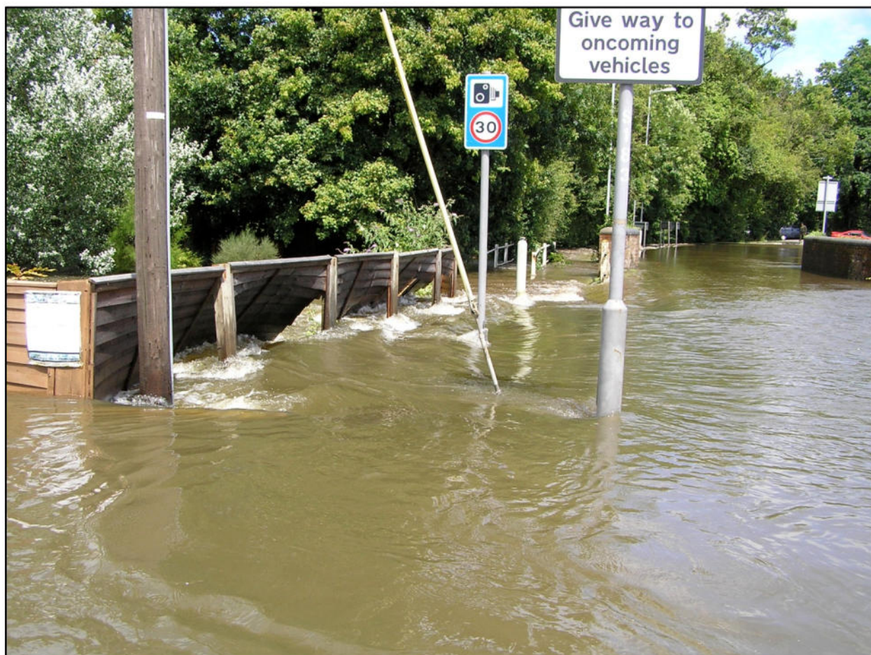
Image 3 (above): the (original) Barkham Bridge under flood, the breached fence of 1 Bridge Cottages being visible.
