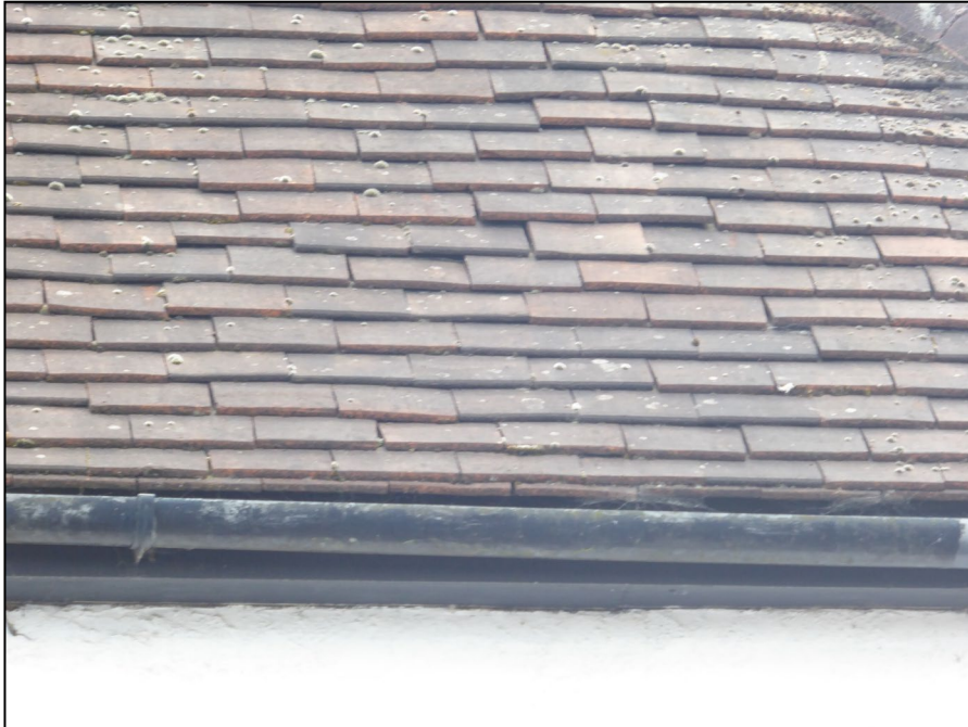
Figure 4. Gaps in roof tiles on north elevation. 75 Pitts Lane, Earley. 05.06.24
