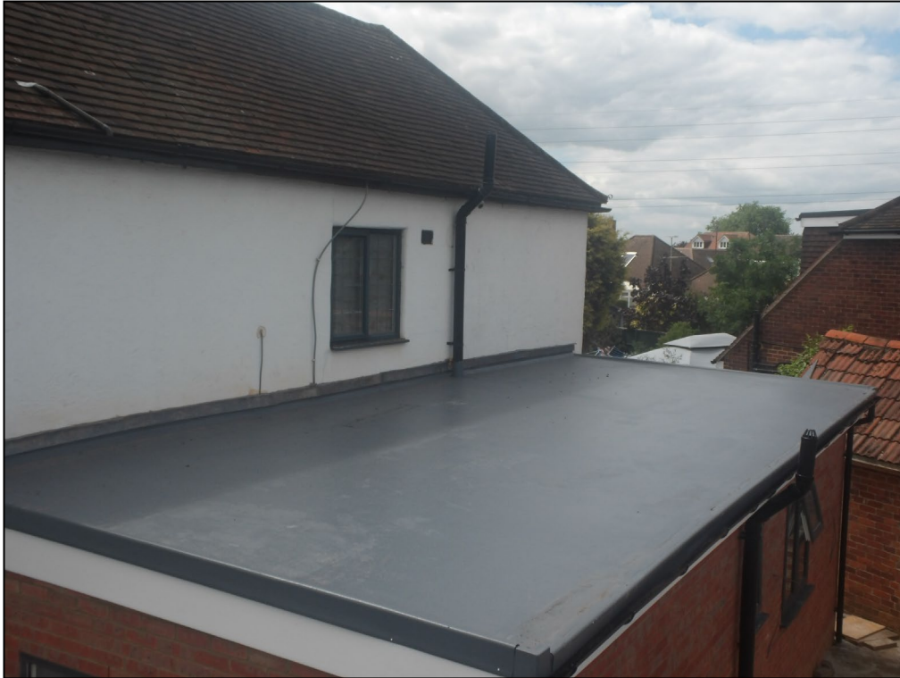
Figure 8. Bitumen felt covering flat roof extension. 75 Pitts Lane, Earley. 05.06.24
