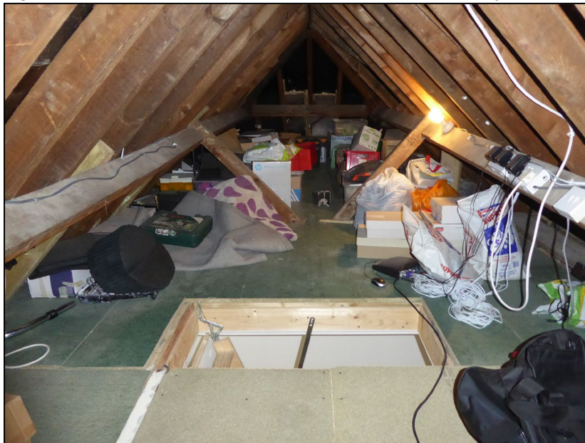
Figure 12. Example of loft space. 75 Pitts Lane, Earley. 05.06.24
