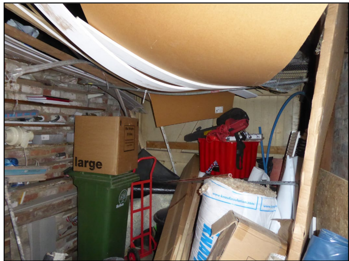
Figure 14. Interior of garage and bitumen lining to tiles. 75 Pitts Lane, Earley. 05.06.24
