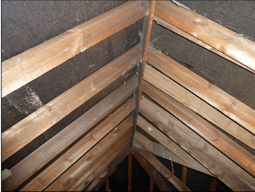
Figure 13. Example bitumen lining in loft. 75 Pitts Lane, Earley. 05.06.24
