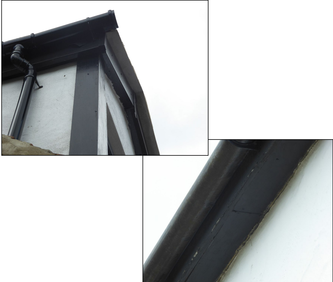
Figure 6. Example sealed soffits and fascias. 75 Pitts Lane, Earley. 05.06.24
