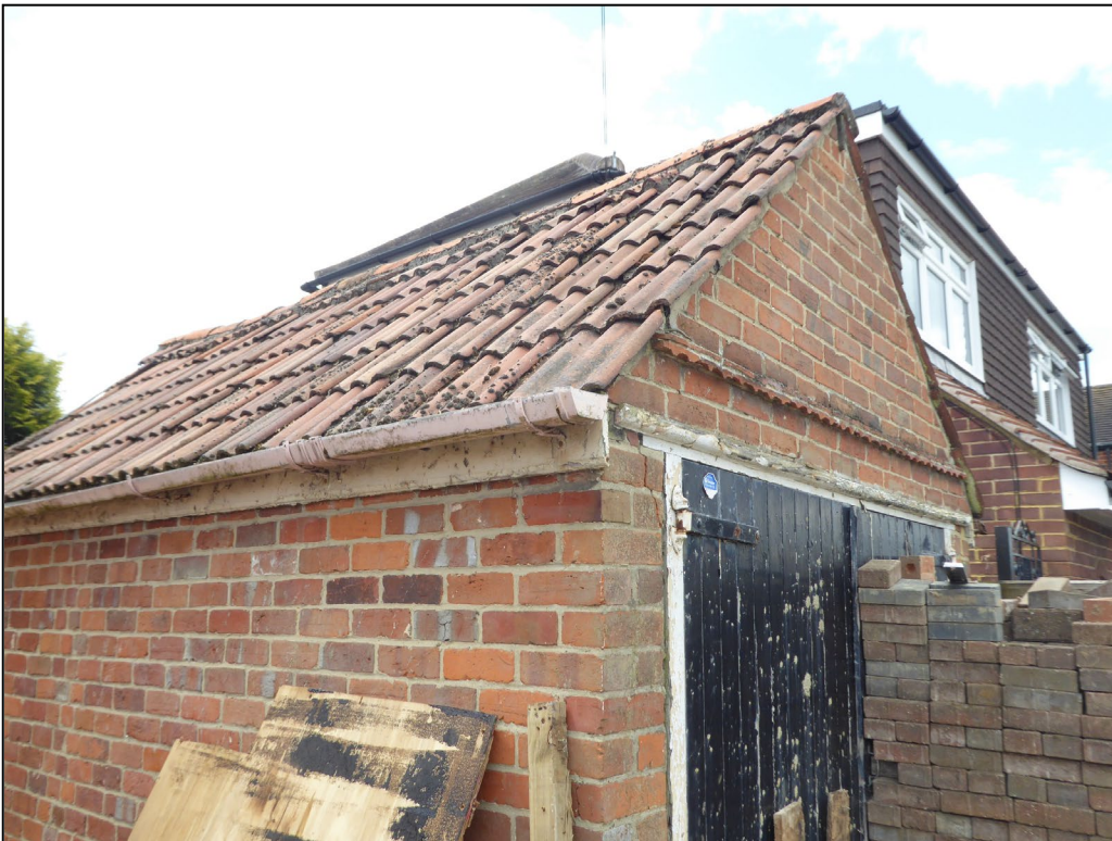
Figure 11. Example roof/ridge tiles, verges and fascia of garage. 75 Pitts Lane, Earley. 05.06.24
