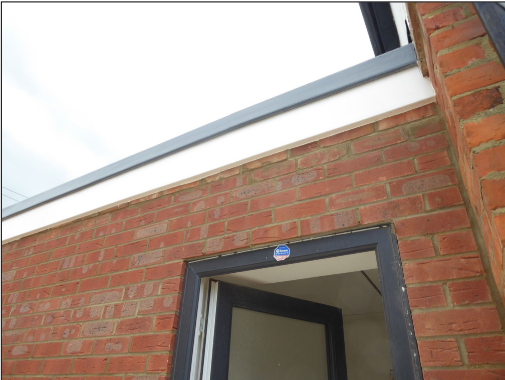
Figure 9. Sealed fascias on flat roof extension. 75 Pitts Lane, Earley. 05.06.24
