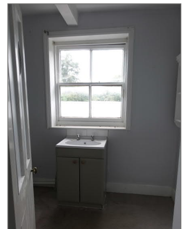
Image 62: View north within C20 extension
