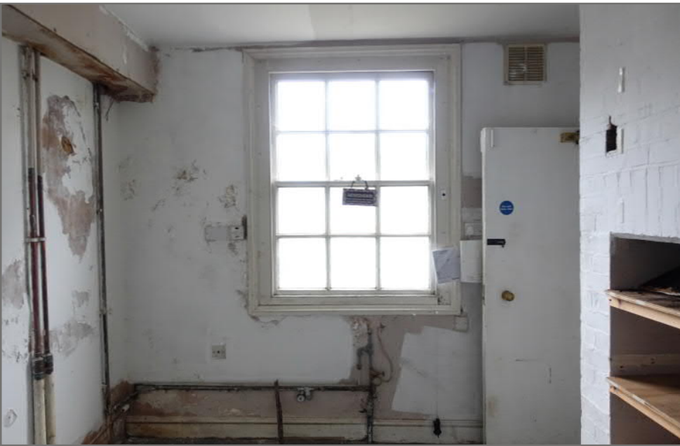
Image 39: View north from C19 extension
