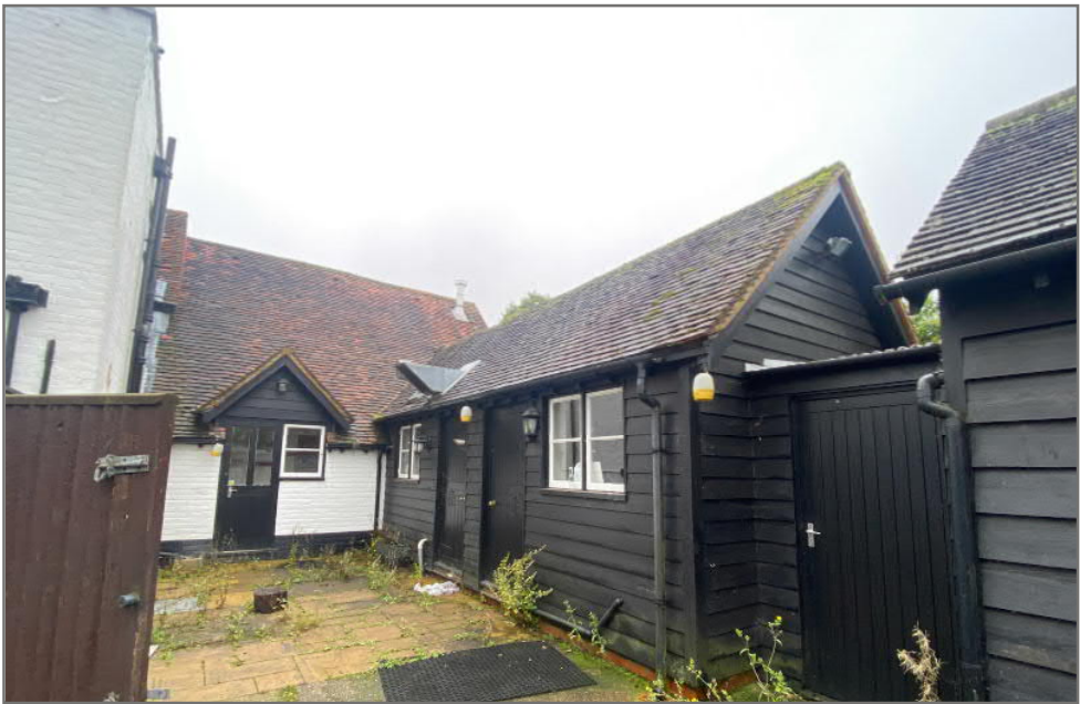
Image 23: View southwest of Kitchen and service yard
