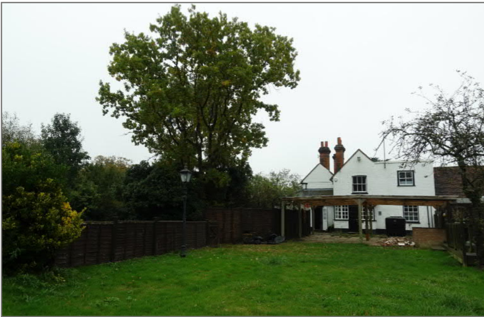
Image 15: View south of north elevation
