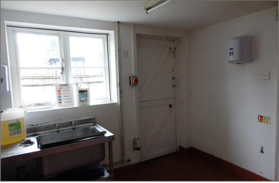
Image 43: View of north extension to Kitchen - door to service yard
