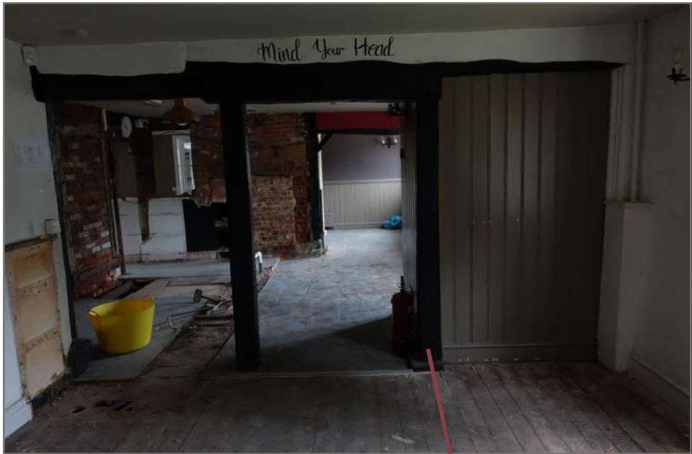
Image 31: View of east towards east room of cottage
