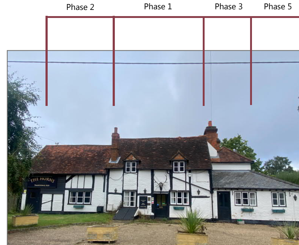
Image 11: South elevation along Crazies Road
