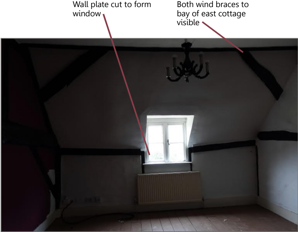
Image 52: View south of east bedroom - modern timber floor and skirting
