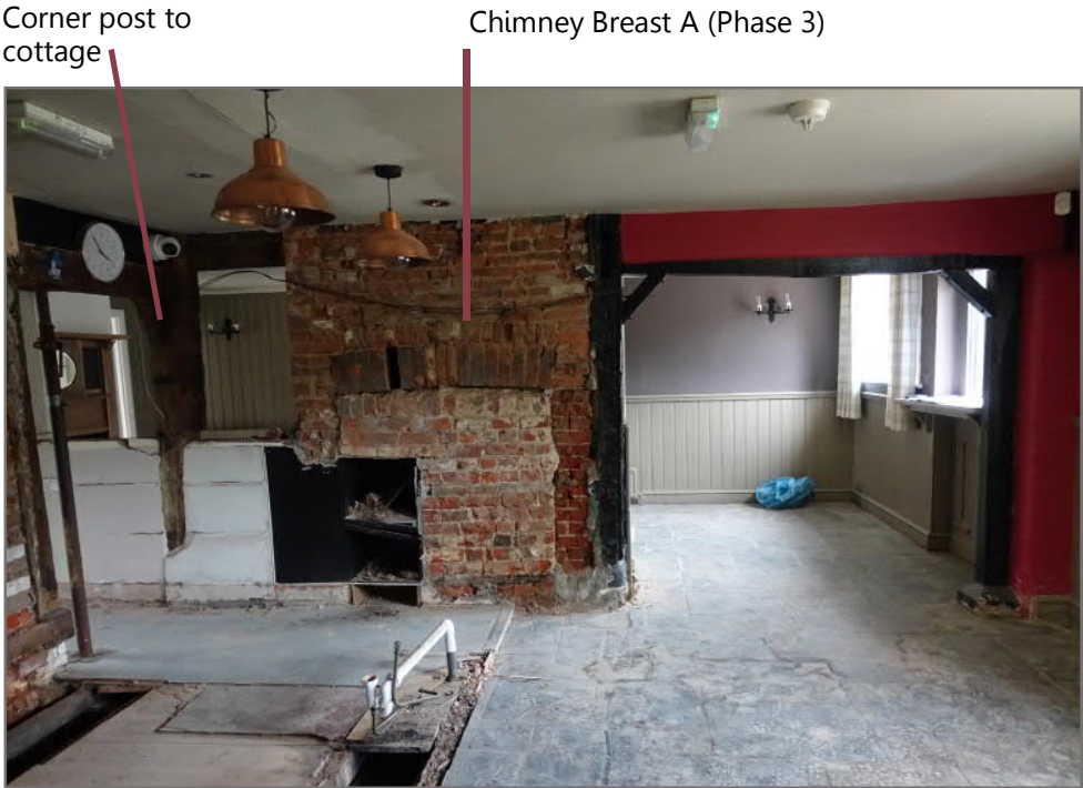
Image 32: View east towards previous external east wall of cottage
