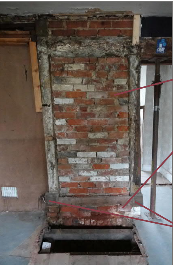
Image 70: View of previous door to be renovated to create an open gap
