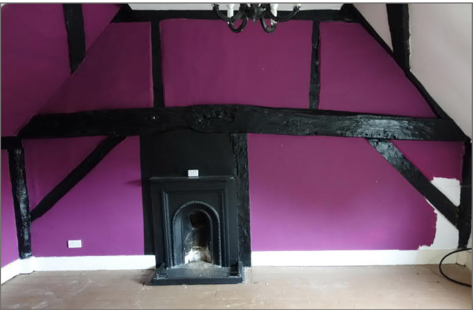
Image 56: View east of east bedroom - possible Edwardian fireplace
