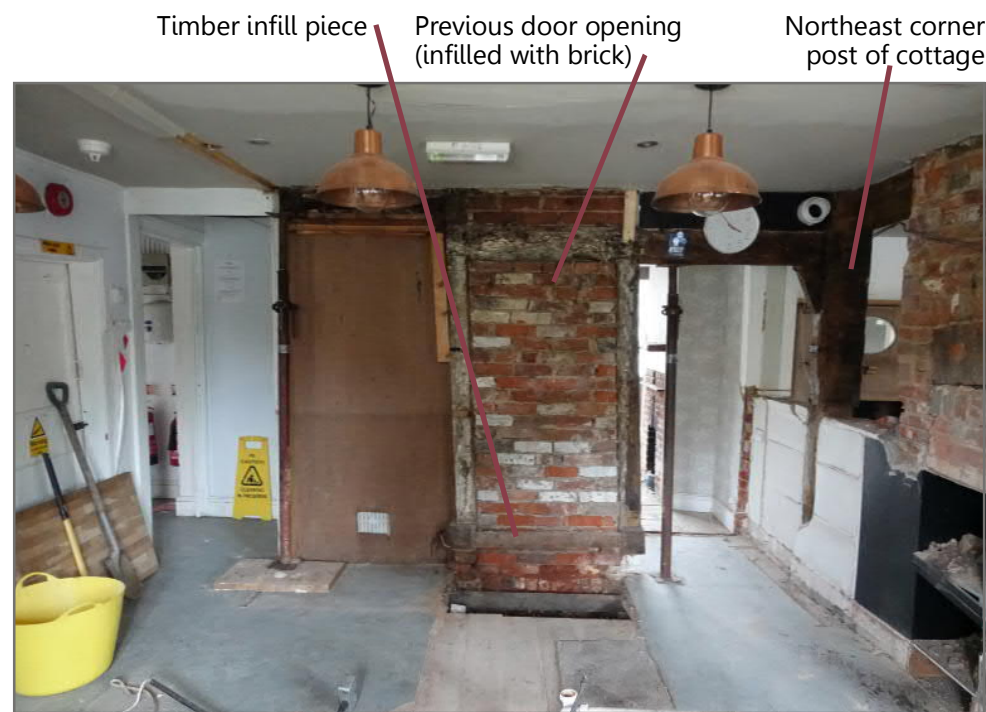
Image 33: View north of previous external wall
