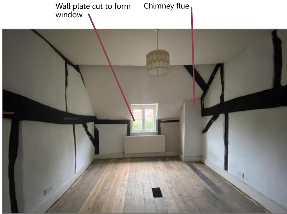
Image 46: View south of west room of C16 cottage - modern timber floor and skirting
