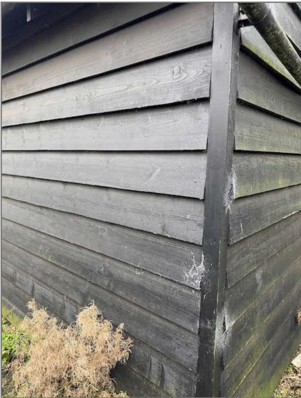
Image 82: Existing timber enclosure - proposed replacement shed to match
