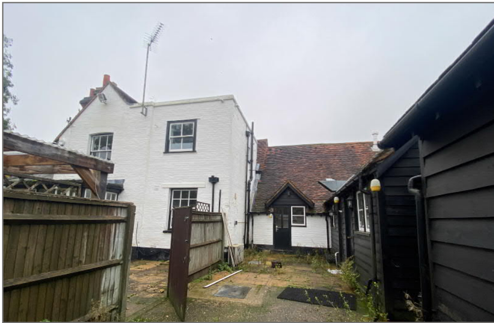
Image 22: North elevation of Barn and service yard
