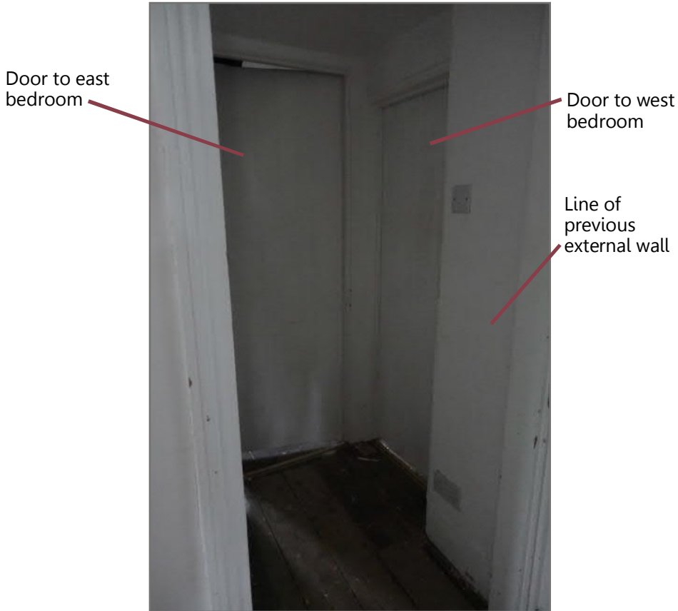
Image 51: View of doors to first floor rooms
