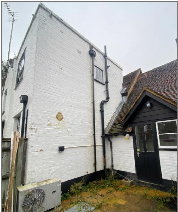
Image 25: West elevation of C20 extension
