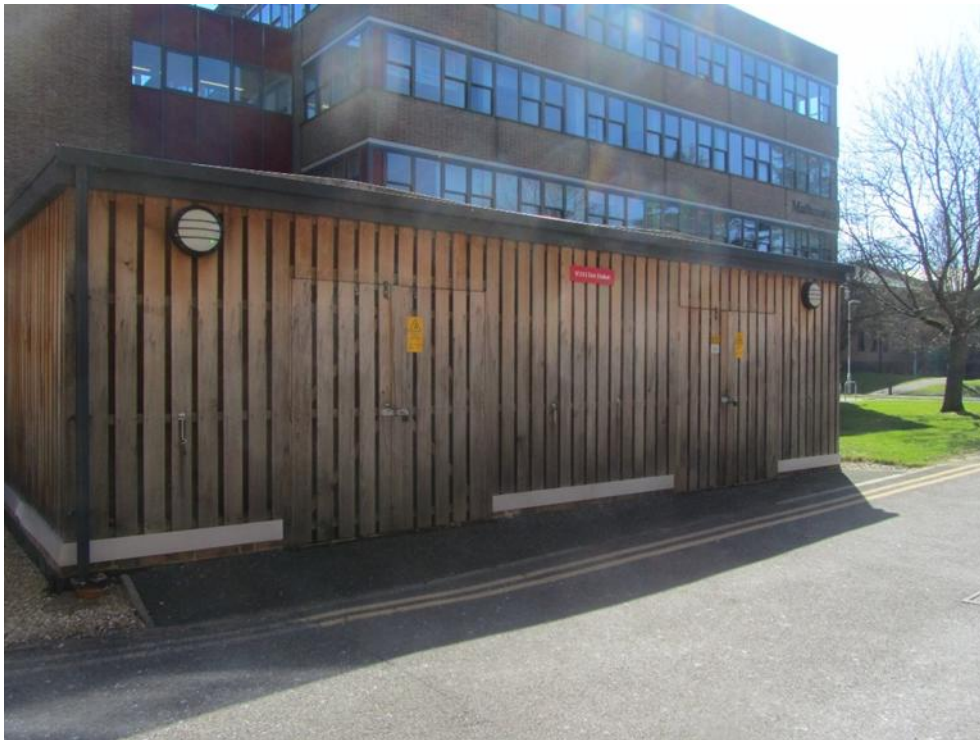
Photo 1 – Front elevation of existing substation
