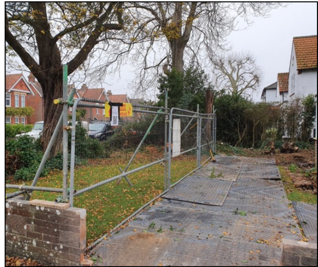
GP2: Tree protection barriers & trackmat ground protection
