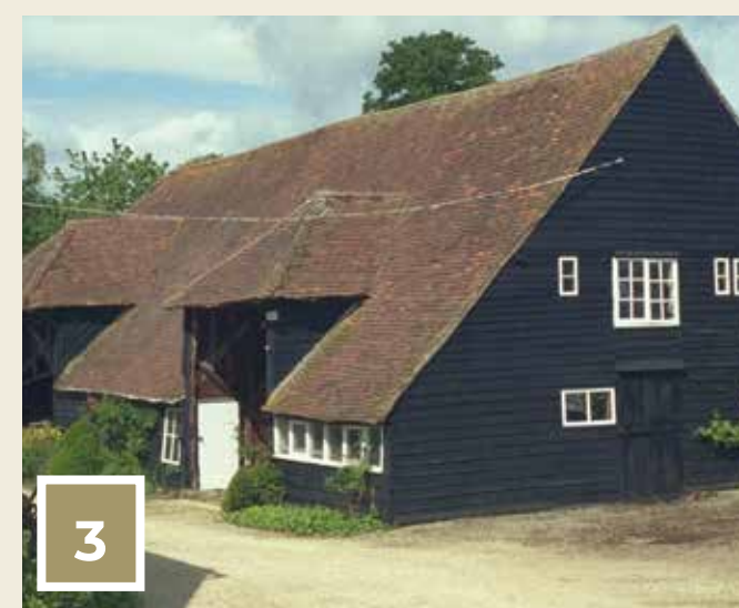
The Barn* (late 17th century) - timber framed, weather boarded and with an old tile roof half hipped
