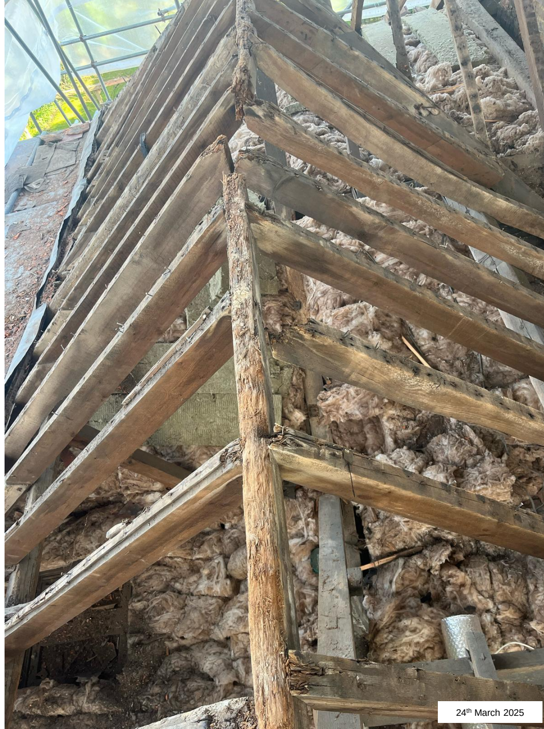
FIGURE 7.5 TYPICAL CONDITION OF RIDGE BOARD AND RAFTERS VIEW LOOKING REARWARDS CURRENT STATE
