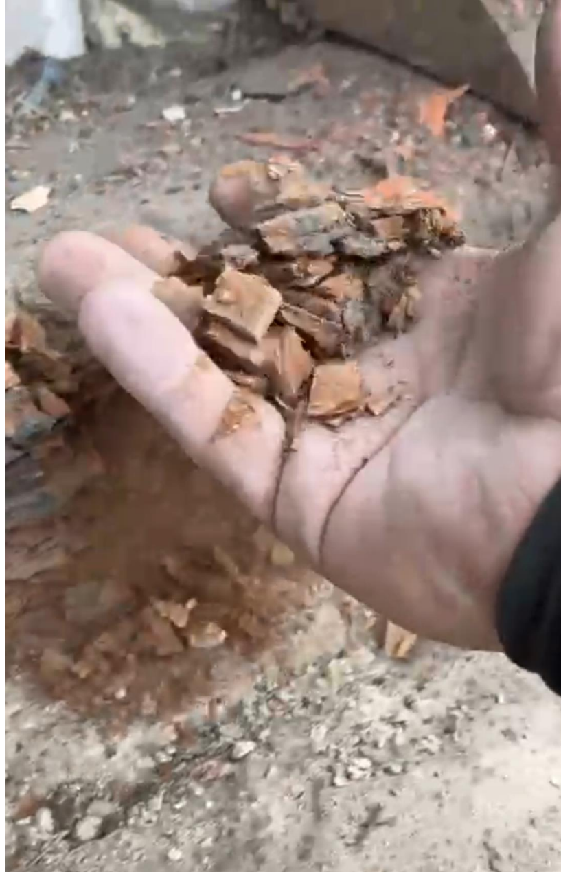
FIGURE 7.13 TYPICAL CONDITION OF WALL PLATE, DISINTEGRATING, CUBOIDAL CRACKING CURRENT STATE (IMAGES TAKEN FROM VIDEO)
