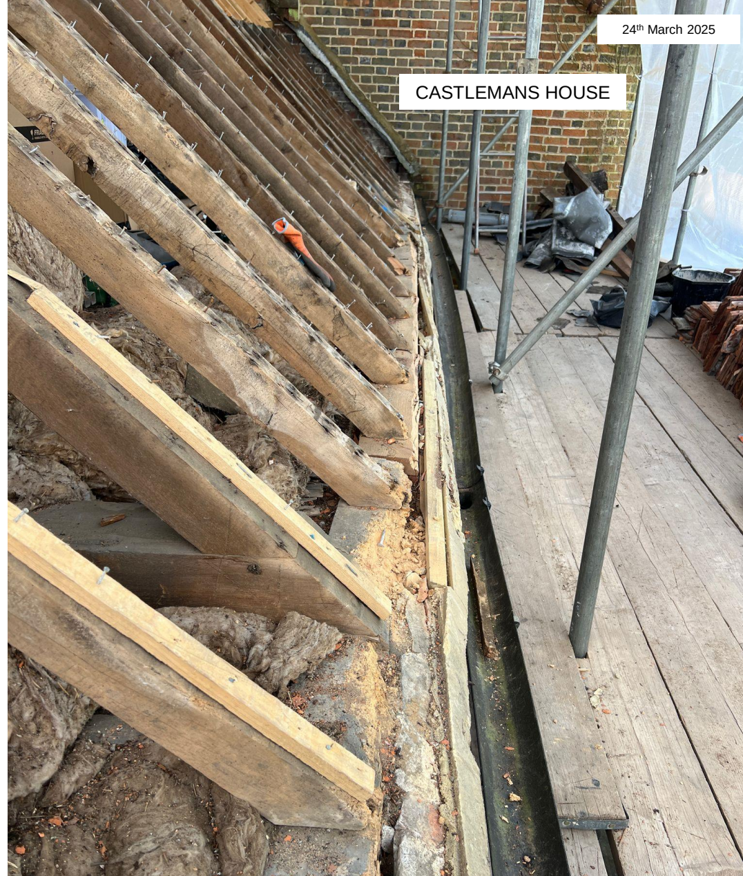
FIGURE 7.11 TYPICAL CONDITION OF WALL PLATE, DISINTEGRATING VIEW LOOKING TOWARDS CASTLEMANS HOUSE, ALONG FRONT ELEVATION CURRENT STATE
