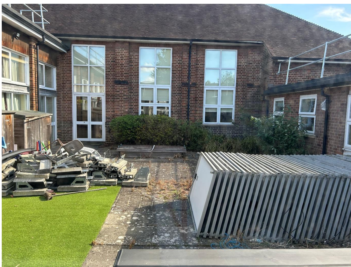
Fig. 5 shows the courtyard of the school as it currently is.
