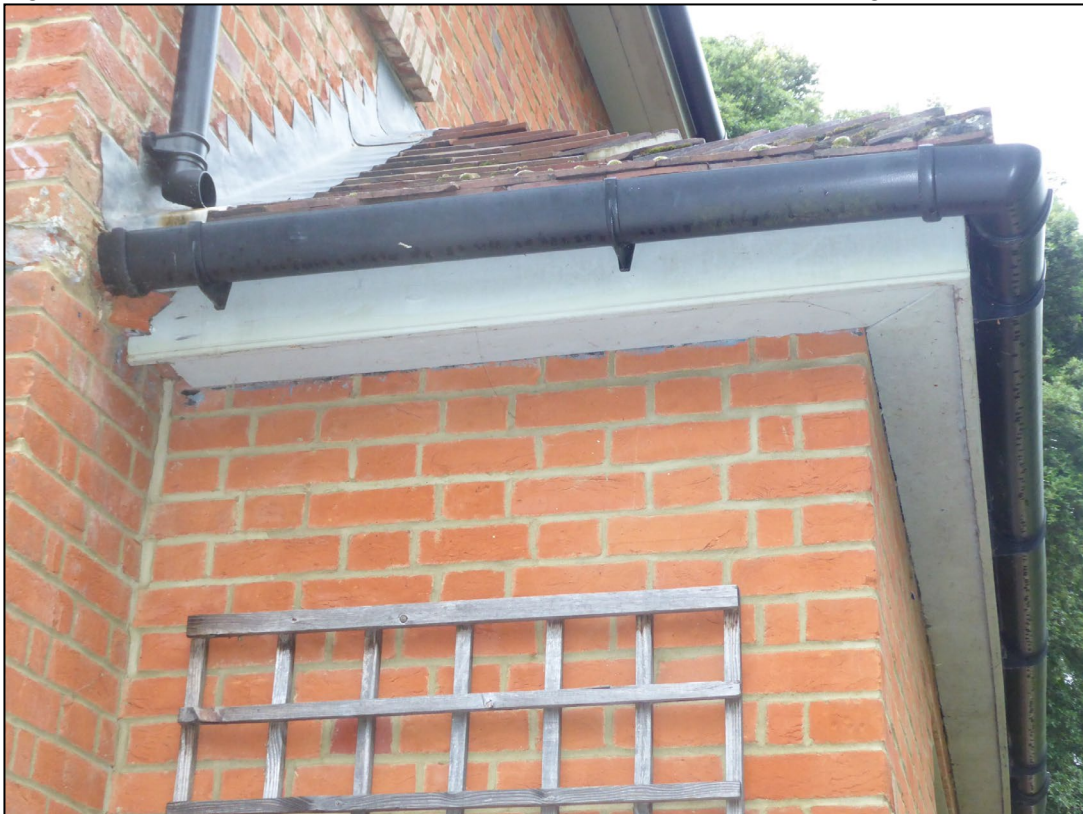
Figure 6. Example sealed soffits and fascias. 8 South Drive, Wokingham. 09.07.24
