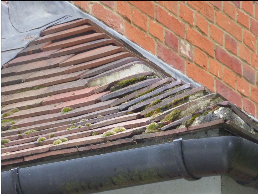
Figure 5. Missing mortar in bonnet tiles. 8 South Drive, Wokingham. 09.07.24
