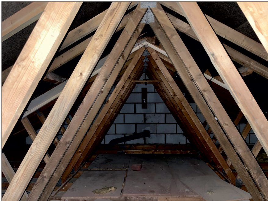
Photograph 3: Showing the attic space.
