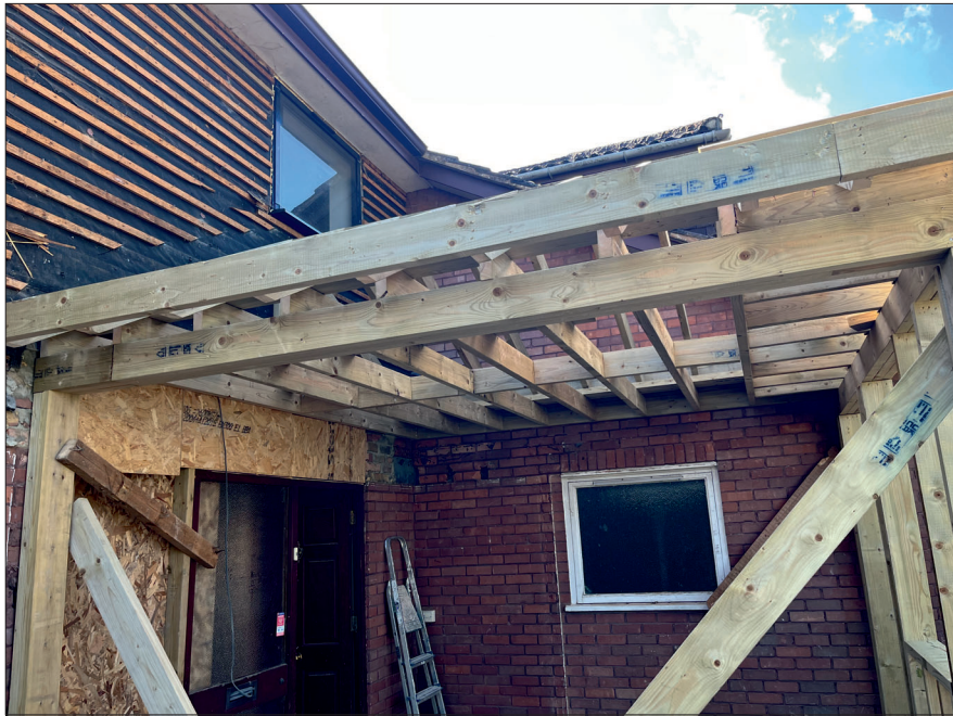
Photograph 1: Showing the timber frame of the new front porch.
