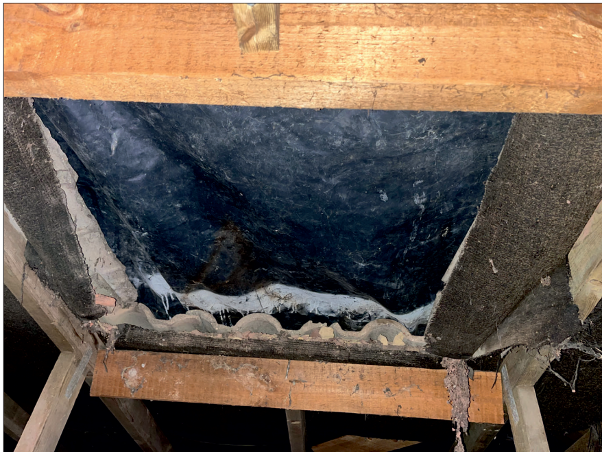
Photograph 4: Showing the area of the removed chimney stack.
