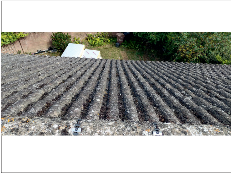
Photograph 2: Showing the well aligned and sealed roof tiles.
