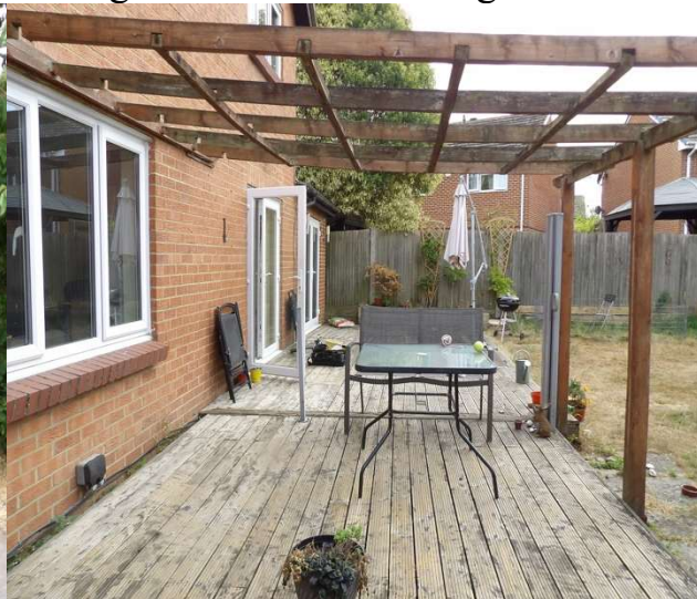
Figure 4. Timber decking to rear.
