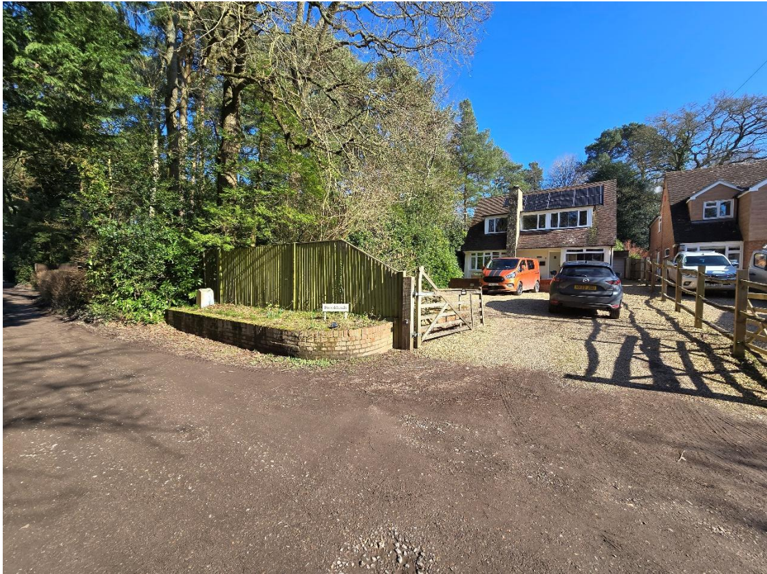
Photo 2 – Low-level brick retaining wall and close board fence to the front of Brooklands
