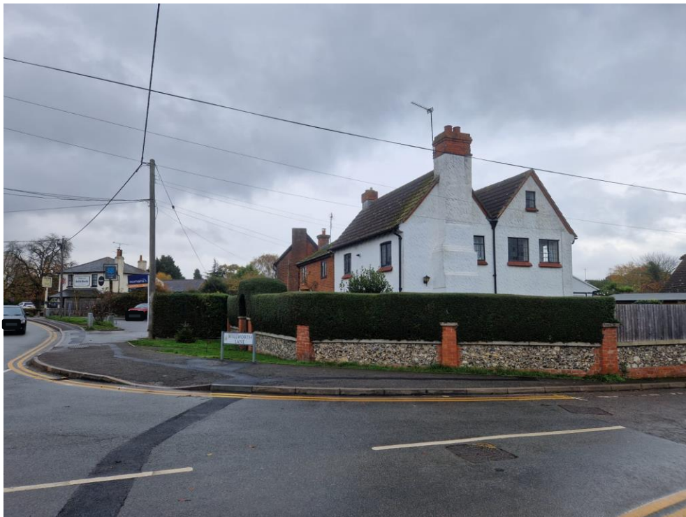
Plate 8: the non-designated Nos. 43 and 45, School Green, viewed looking north-east.
