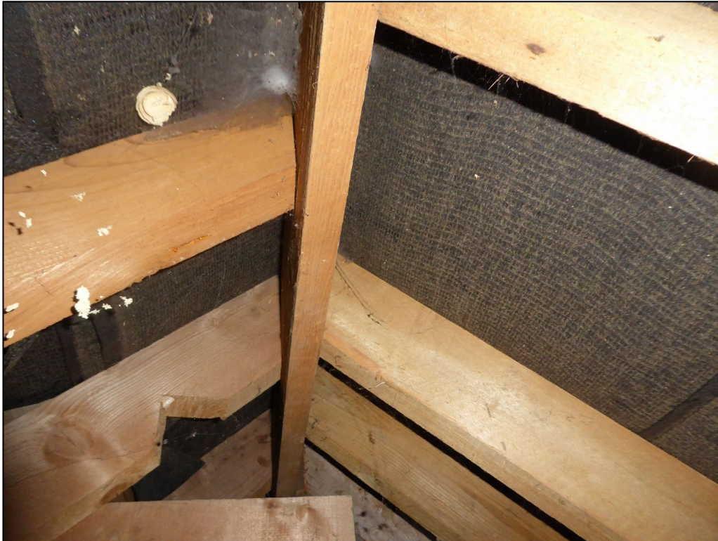
Figure 10. Example tile lining. Rose Cottage, Limmerhill Road, Wokingham. 09.07.24
