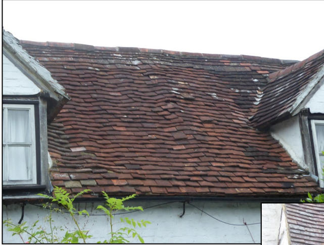
Figure 5. Example cracked/slipped/raised roof tiles. Rose Cottage, Limmerhill Road, Wokingham. 09.07.24
