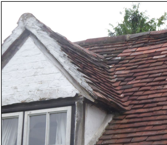
Figure 6. Example sealed verges. Rose Cottage, Limmerhill Road, Wokingham. 09.07.24
