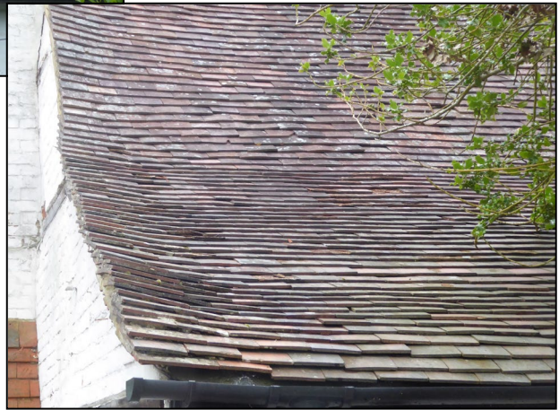
Figure 6. Example sealed verges. Rose Cottage, Limmerhill Road, Wokingham. 09.07.24
