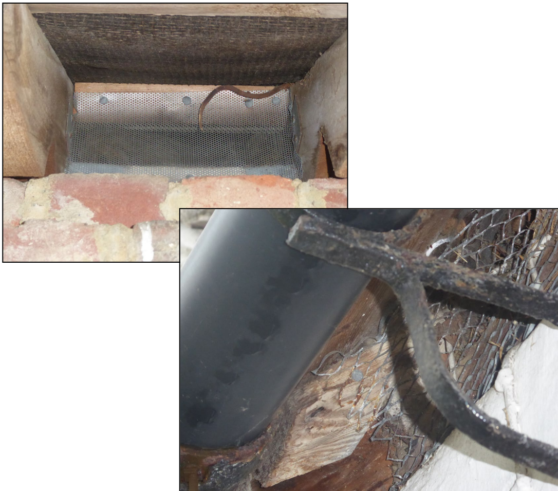
Figure 8. Example sealed eaves. Rose Cottage, Limmerhill Road, Wokingham. 09.07.24
