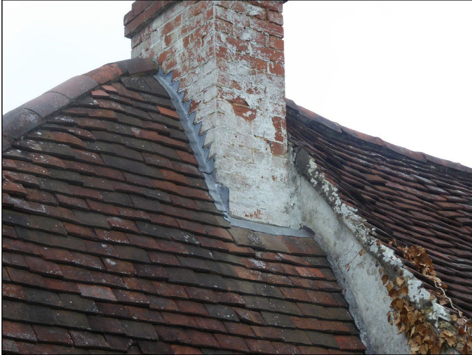
Figure 7. Example sealed lead flashing. Rose Cottage, Limmerhill Road, Wokingham. 09.07.24
