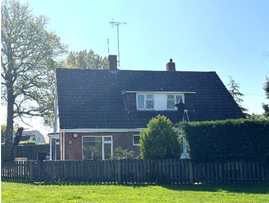
Photograph 1. Chalet bungalow viewed from the north.
