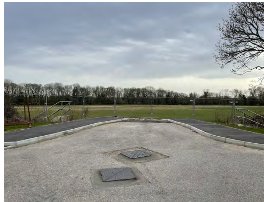
VIEW OF SECONDARY ACCESS INTO THE SITE
