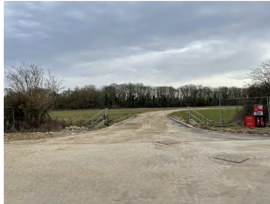
VIEW OF PRIMARY ACCESS INTO THE SITE
