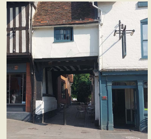
Figure 71: Typical covered passageway leading to courtyard
