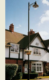
FIGURE 214 PRIMARY ROUTE LIGHTING COLUMN & LANTERN
