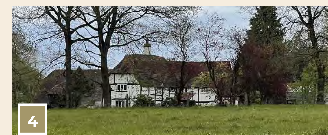
The Farmhouse (15th century) is an L-shaped hall house, timber framed with painted brick infill, old tiled gabled and half hipped roof
