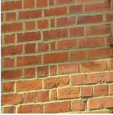
Red Facing Brickwork at ground floor level (to match existing)
