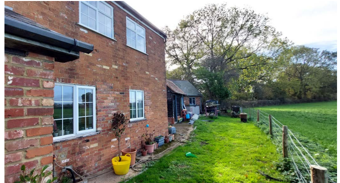
Figure 17. Rear Elevation of Damsonwell
