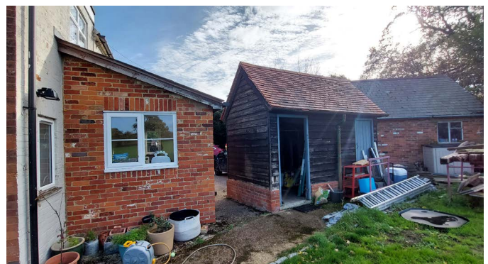
Figure 20. Single-Storey Extension and Outbuildings
