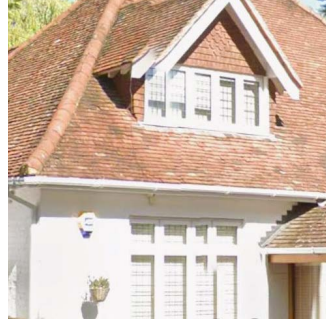
White Painted Brick and Clay Tile Roof
