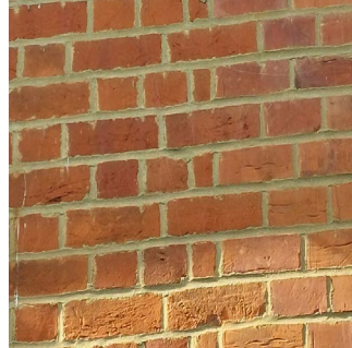
Red Facing Brickwork
