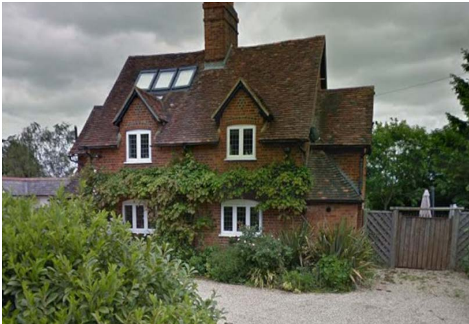
Figure 10. Carrington Cottage, Wokingham Road (Google Maps)
