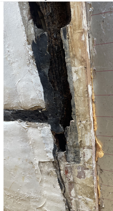
Remains of lower portion of southern principal post.
