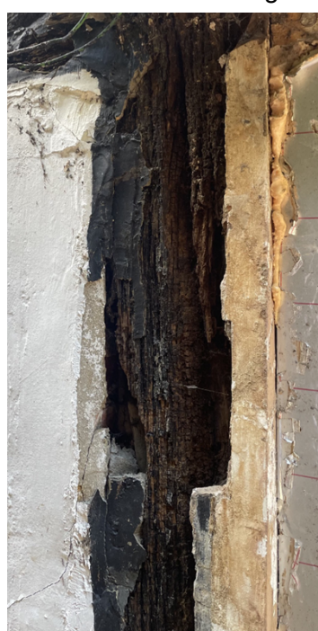
Remains of lower portion of southern principal post.
