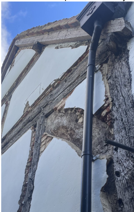
Revealed brace timber.
