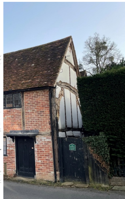
West Gable End – phot shows the braces have now been exposed
