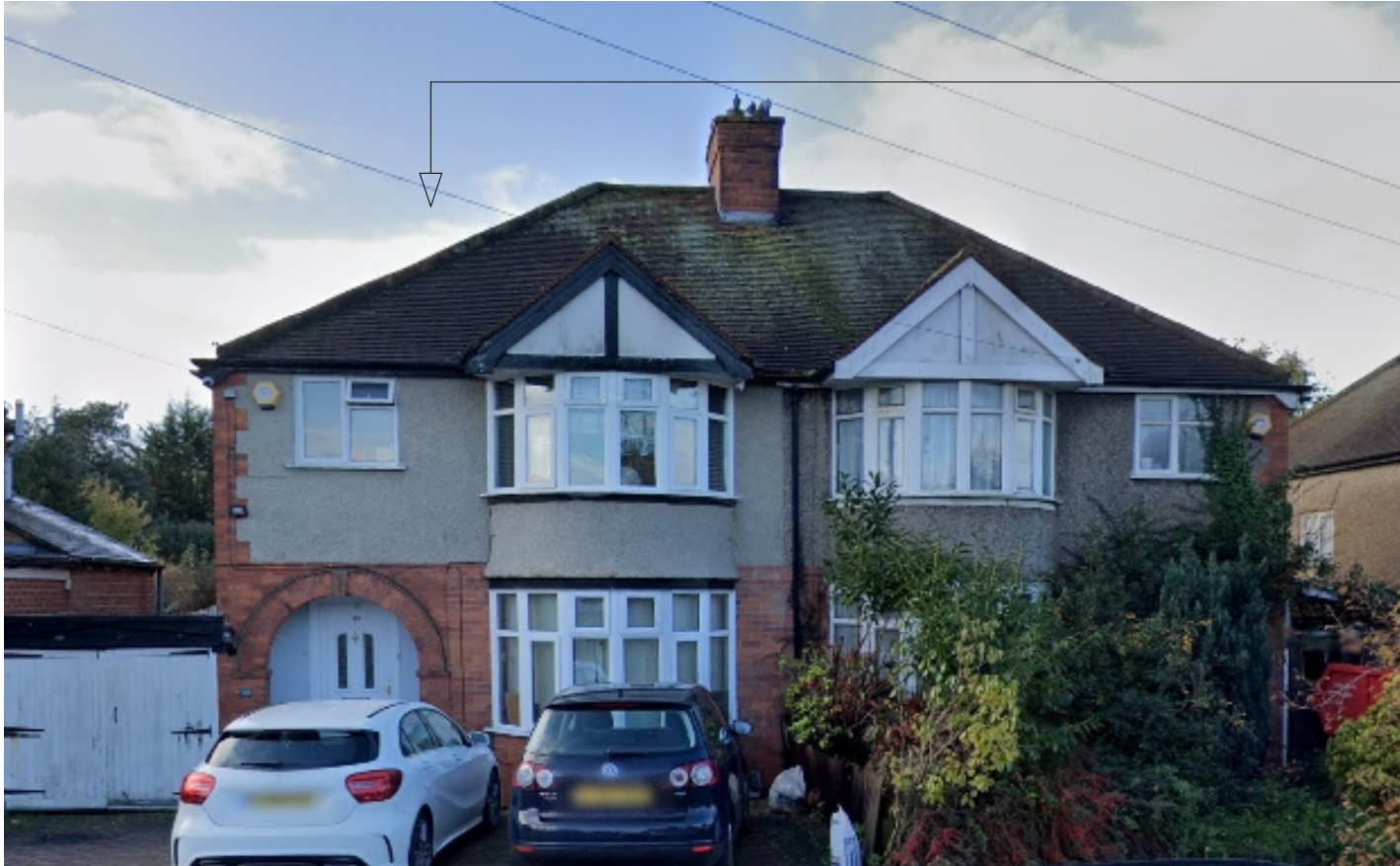
EXISTING FRONT PHOTO VIEW - 01 SCALE - N T S A001
