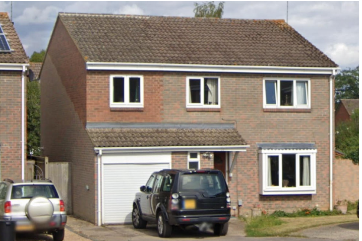
Local precedent: extension above garage, ridge line carried through, Kestrel Way.
