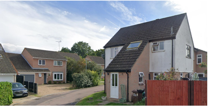
Local precedent: render finish in street scene (opposite site), Kestrel Way.
