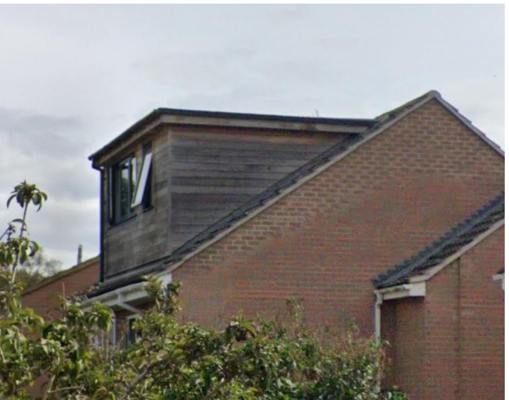
Local precedent: roof height raised and dormer extension, Starling Way.
