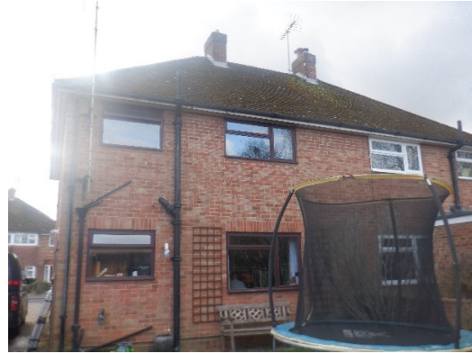
Photograph 2. Rear of the house viewed from the east.
