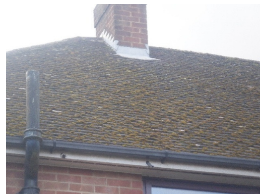
Photograph 6. Lead flashing tight around the chimney.
