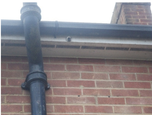
Photograph 5. Sealant present along the soffits at the eaves.
