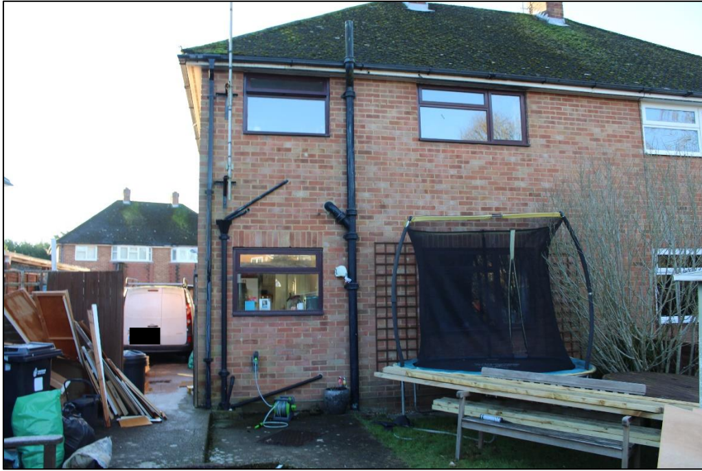
Photograph 2 – Rear elevation as viewed from the garden
