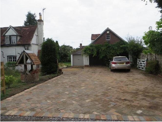
Front driveway and parking.
