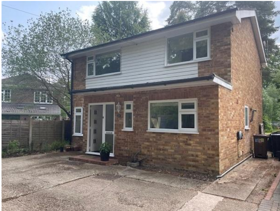
21 Sandhurst Road Front North East/Side North West
