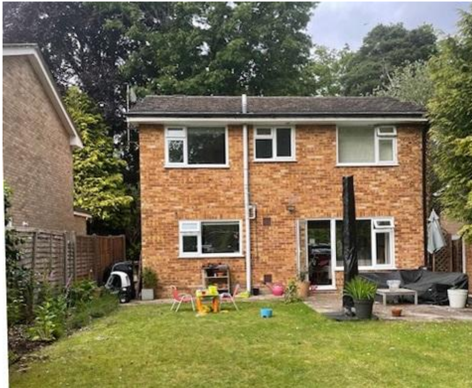
21 Sandhurst Road Rear South West
