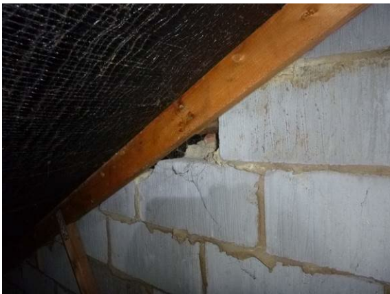
Photograph 12. Gap over gable blockwork (roof void).
