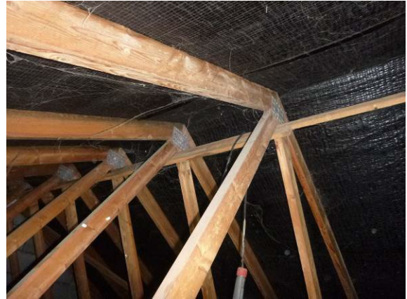
Photograph 11. Cobwebbed ridge (roof void).
