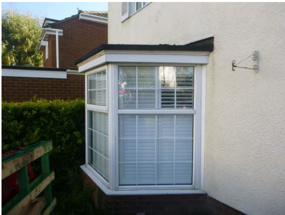
Photograph 6. Tight bituminous roofing felt on the bay window (front elevation).
