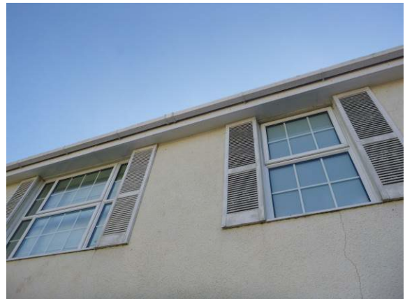
Photograph 7. Shutters tight to the rendered walls (front elevation).
