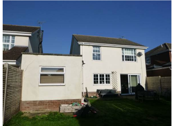
Photograph 2. Rear of property viewed from south.
