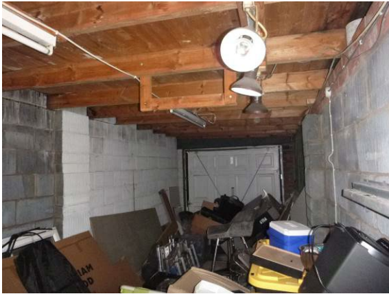
Photograph 14. Internal view of the front northern end of the garage..
