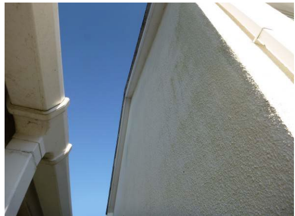
Photograph 4. uPVC soffits on gables (western elevation).
