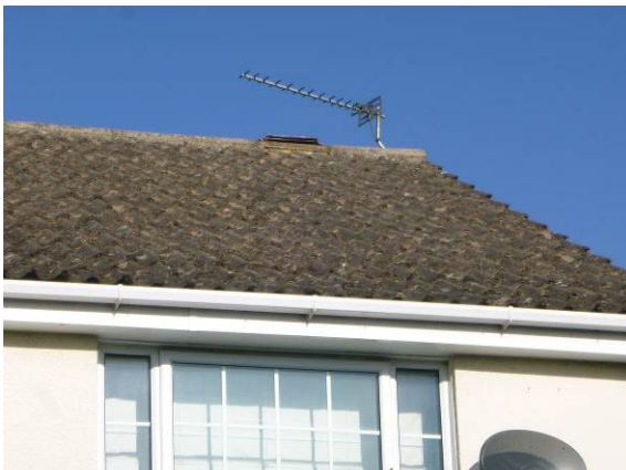
Photograph 3. Interlocking roof tiles and intact ridge tiles (rear elevation).
