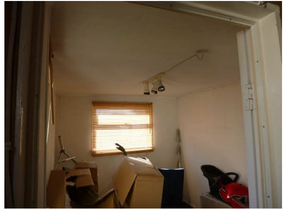
Photograph 15. Rear southern end of the garage with plastered walls. .
