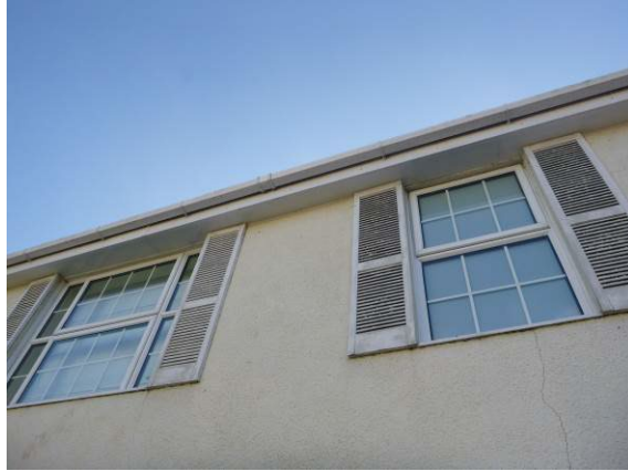
Photograph 5. uPVC soffits at eaves (front elevation).
