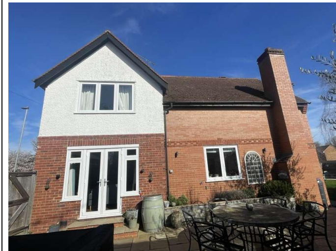
The southern elevation of B1
