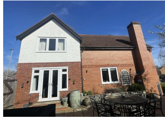
Photo 2: The southern elevation of B1
