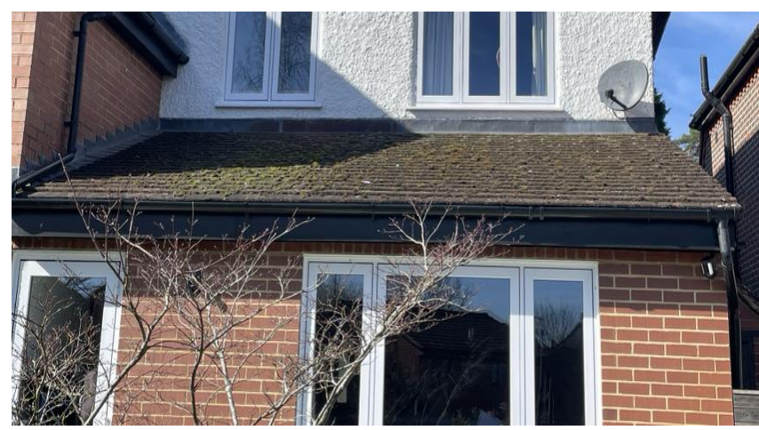
Photo 4: Single storey extension which will be affected by the development
