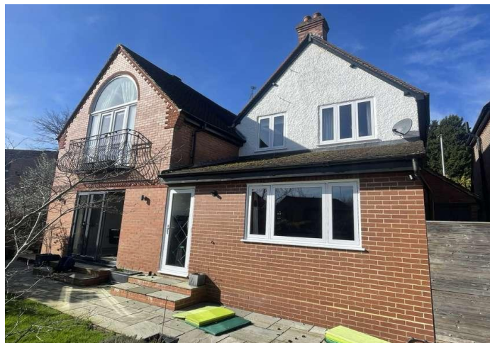
Photo 3: The eastern elevation of B1
