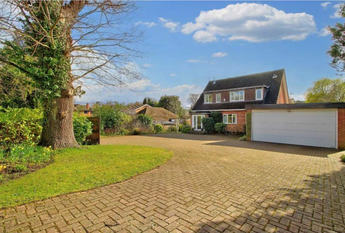
PIC 1- FRONT OF THE HOUSE
