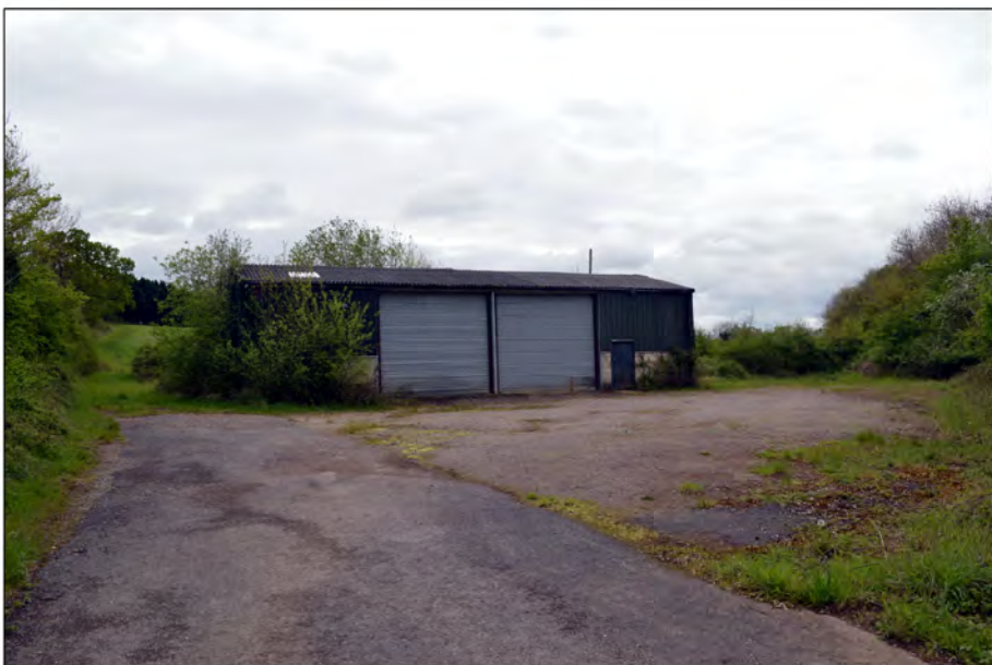
Photo 2) Storage building and yard at the northern end of the Site, viewed from the north
