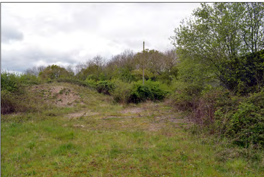
Photo 3) Bund to the rear (south-east) of the storage building
