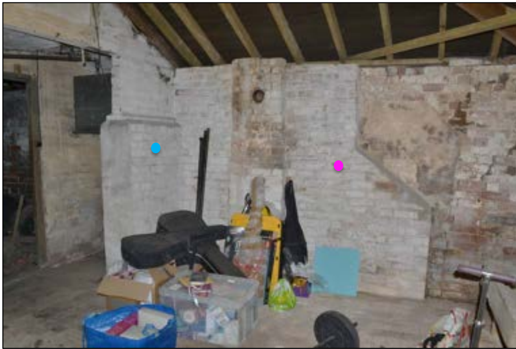
Figure 50: Main store, first room of the outbuilding you enter upon exiting the utility/pantry, (left) note remnants of the original dividing wall highlighted in blue and evidence of a flue/chimney at one point in time highlighted in pink, (right) door that leads into 20 th century link between the outbuilding and principal house
