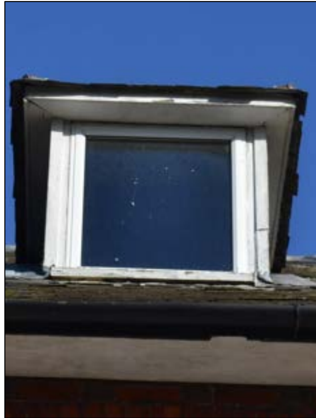
Figure 20 - Details of windows on the south elevation (left) inappropriate 20 th century uPVC top hung casement window, (centre) dormer window thought to originally house the clock when the house was briefly a school. (Right) Original timber single glazed leaded window - internally there is secondary glazing behind it. Note both windows (left and right) have flat segmental arches above
