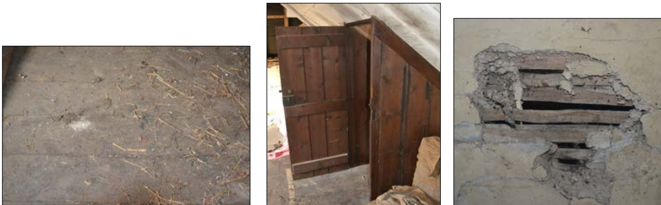
Figure 25: Attic room details (left) solid timber floor, (centre) timber door leading to stairs to access the ground floor, (right) exposed historic lath and plaster
