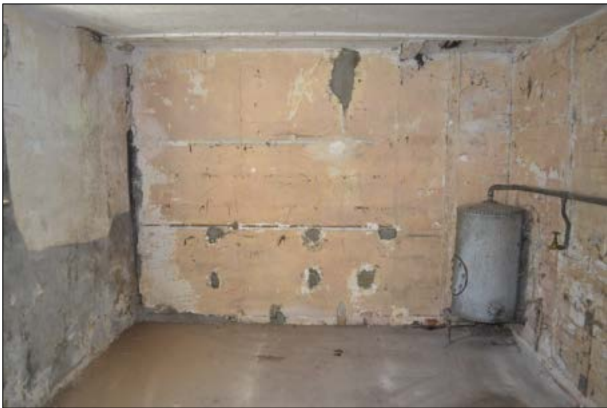
Figure 53: Internal view of boiler room- note (left) the evidence of the later timber frame and brick infill wall visible through the plaster/render. The concrete floor is a later 20 th century addition
