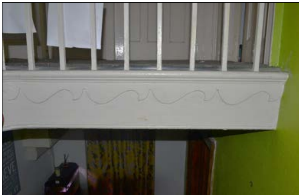
Figure 33 - Details of early 19 th century staircase, note the stick balusters, mahogany banister, and carved brackets under the treads
