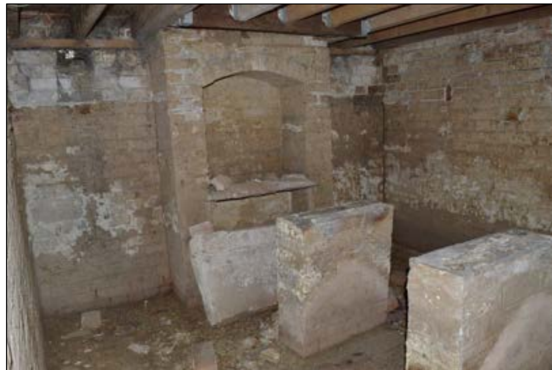
Figure 46: Cellar rooms - note the walls are brick lined and there are recessed oven arches
