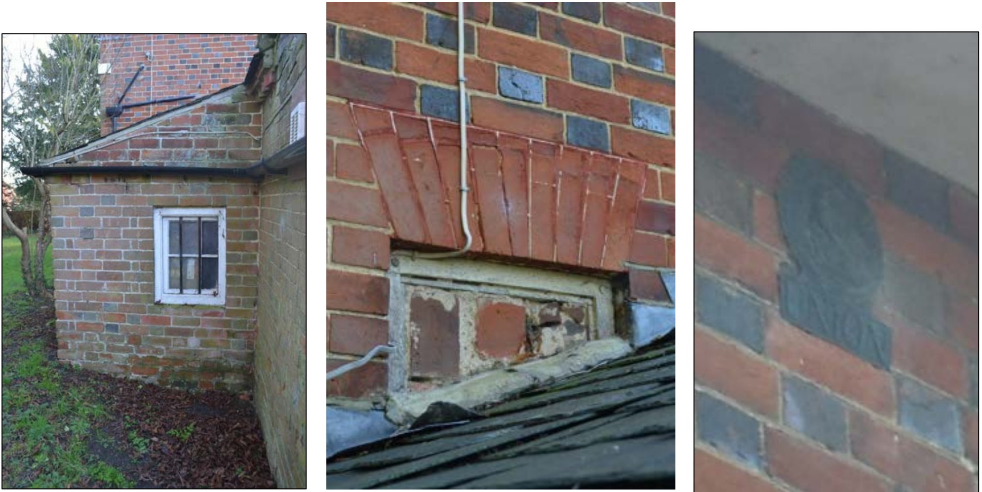
Figure 22: Details of the west elevation- (left) 20 th century link extension attaching the outbuilding to the principal building, (centre) blocked off window which would have originally opened into what is now the kitchen, (right) iron plaque under the eaves - date unable to be read from ground level or images, however, the word 'UNION' can be clearly seen.
