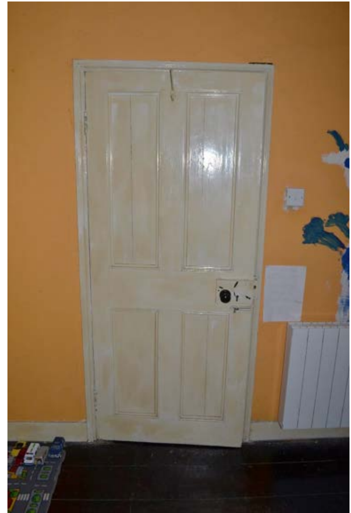
Figure 29: Bedroom one - note the solid wood exposed floor and 4 panelled timber doors. (left) door leads into Bedroom three - thought to be a later alteration
