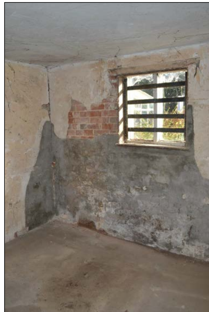
Figure 53: Internal view of boiler room- note (left) the evidence of the later timber frame and brick infill wall visible through the plaster/render. The concrete floor is a later 20 th century addition
