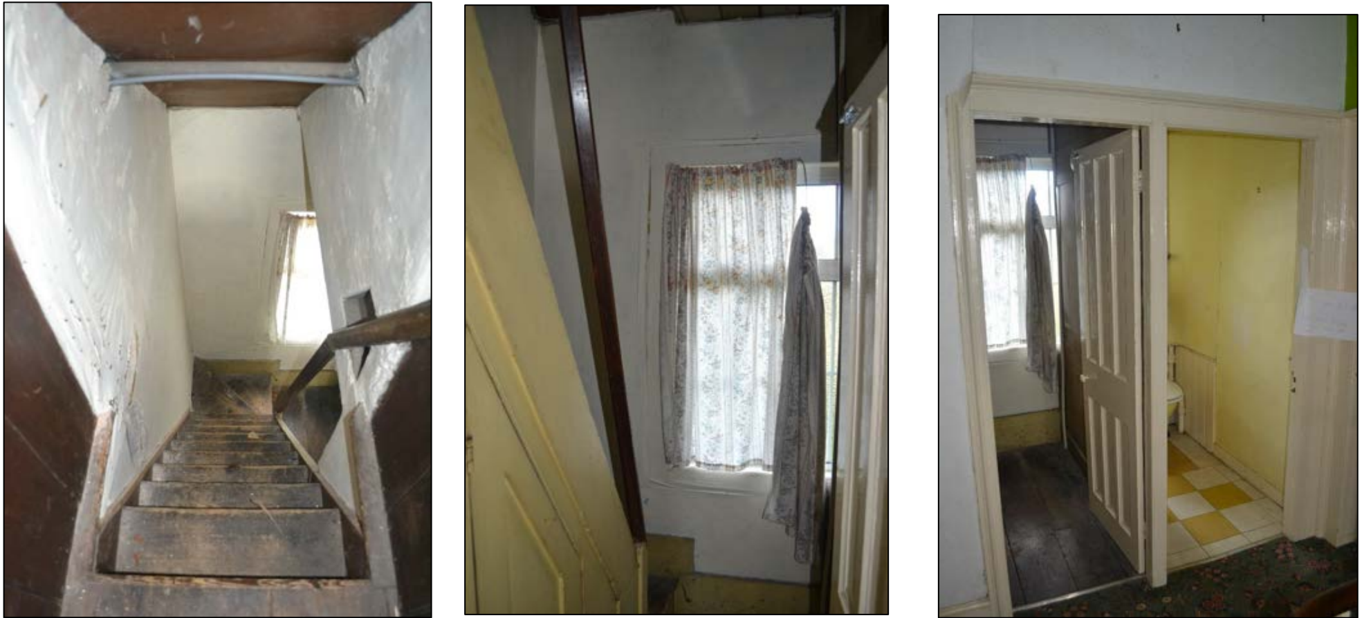
Figure 26: (left) steep timber stair leading from attic room to ground floor, (centre) window that is cut through on the ground floor to accommodate stud partition wall, (right) stud partition wall- later 20 th century addition to allow the insertion of a toilet
