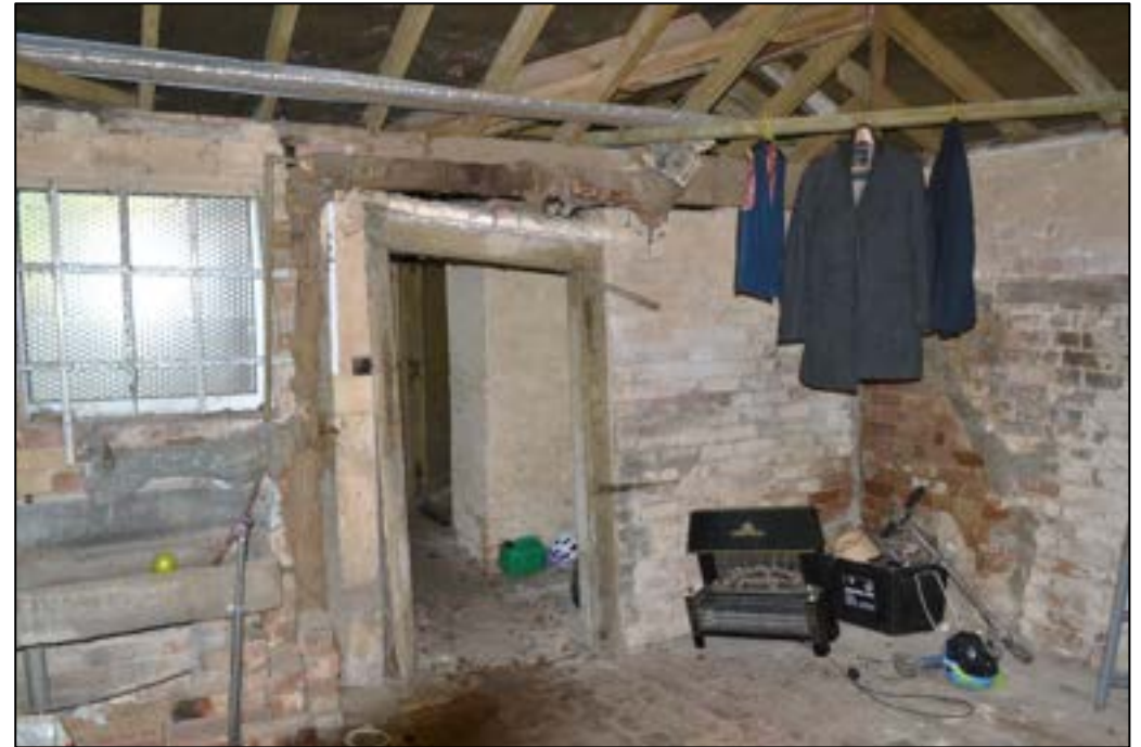
Figure 50: Main store, first room of the outbuilding you enter upon exiting the utility/pantry, (left) note remnants of the original dividing wall highlighted in blue and evidence of a flue/chimney at one point in time highlighted in pink, (right) door that leads into 20 th century link between the outbuilding and principal house
