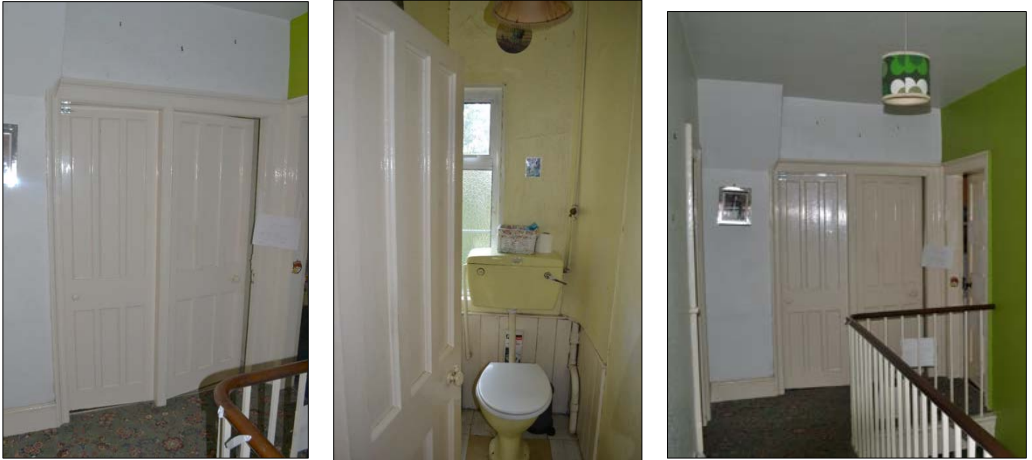
Figure 27: (left) 19 th century doors accessing the attic rooms and toilet taken from the ground floor sitting room and kitchen, (centre) later 20 th century toilet, (right) hallway leading to rooms at the front of the house, toilet, and attic room
