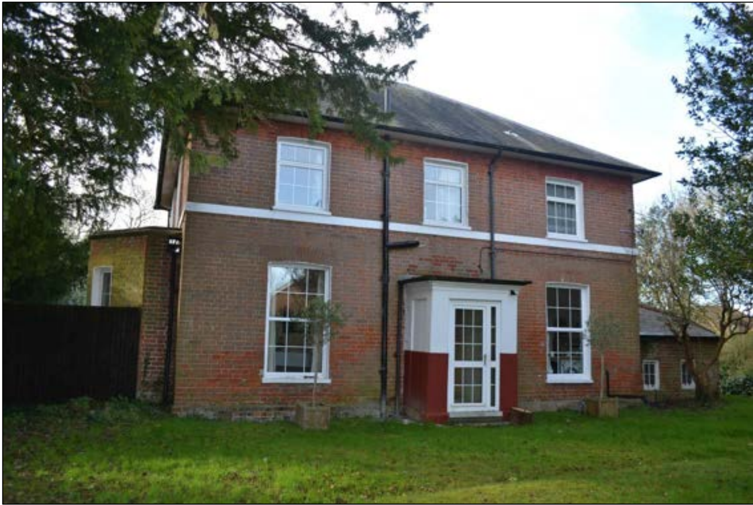
Figure 14: North (front) elevation of Sussex Lodge
