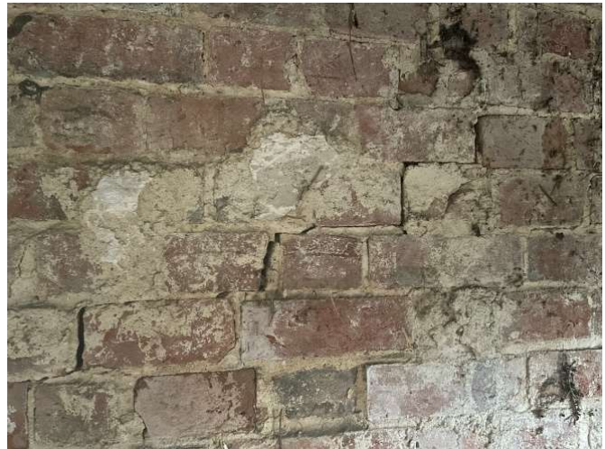
B - Cracks internally and externally - areas of diagonal cracking, significant vegetation/root damage, making good historic repairs
