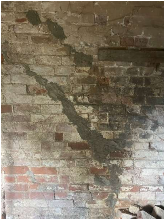
B - Cracks internally and externally - areas of diagonal cracking, significant vegetation/root damage, making good historic repairs
