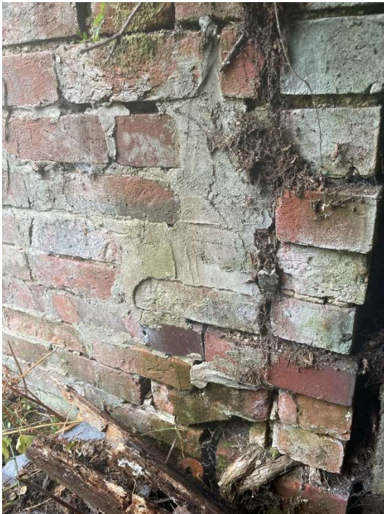
C - Blown bricks - to be replaced/turned
