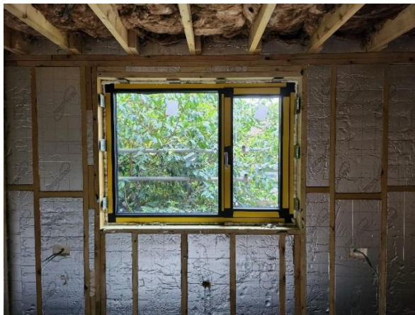
Fig 1. Reinstated window looking out towards 12 Heatherway
