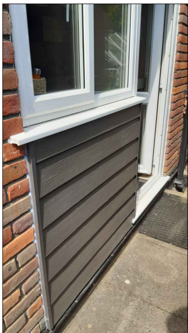
Existing cladding under window
