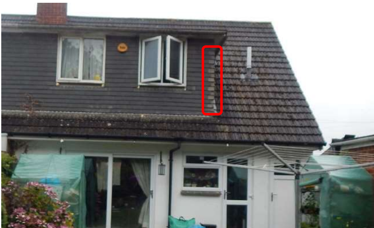
Image 2 – Front North facing elevation of the property offering gaps of adequate proportions within the vertical hanging tiles of value to bats for daytime roosting
