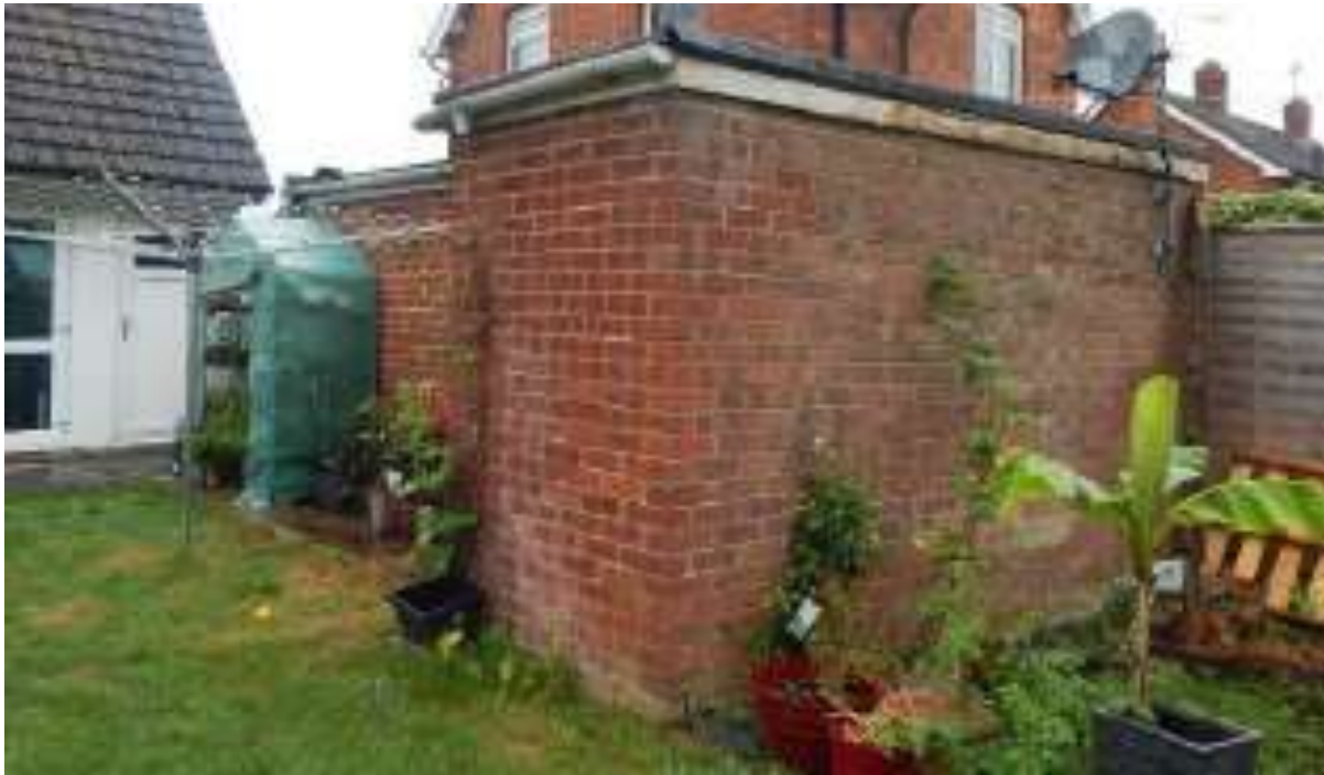
Image 7 – Detached brick garage structure to the rear of the property which has demonstrated no features of value to bats
