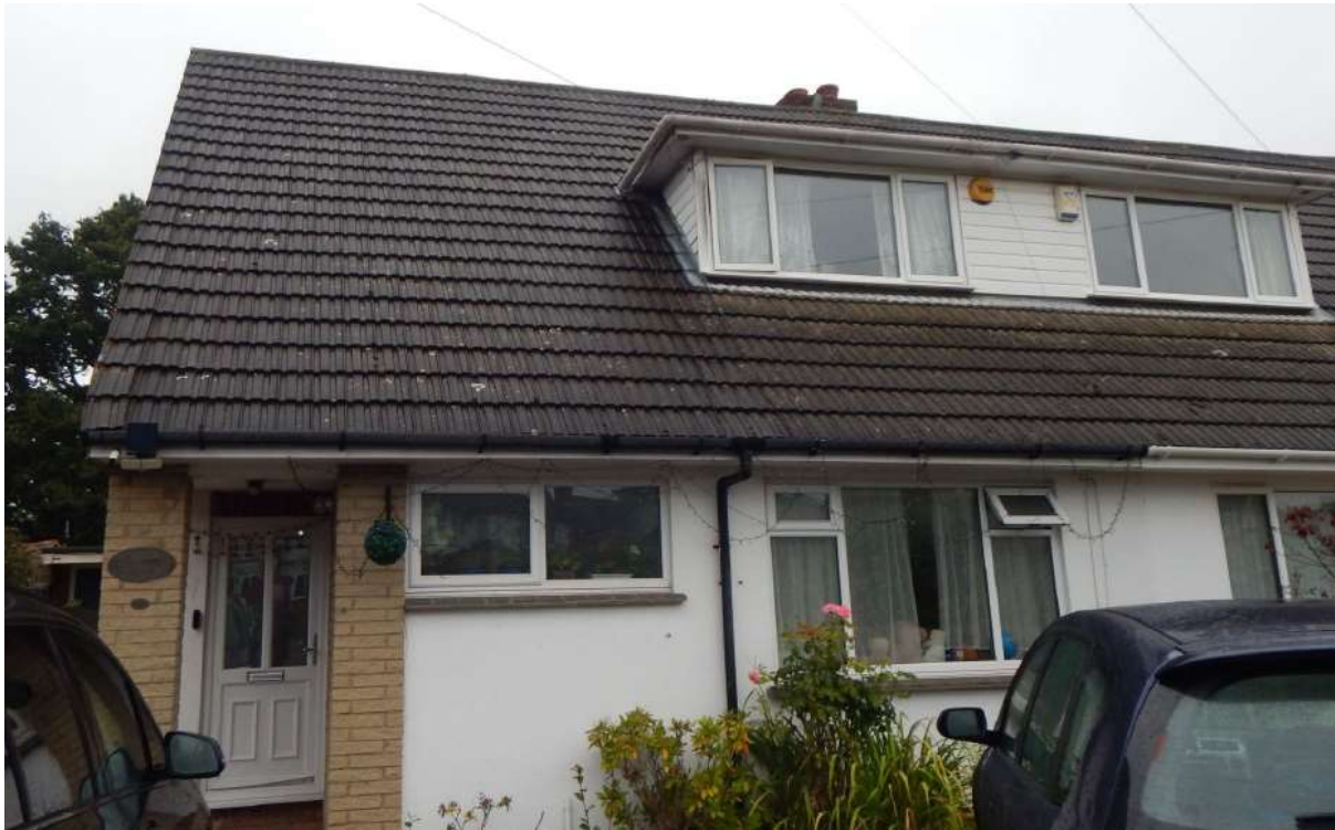
Image 1 – Front South facing elevation of the property
