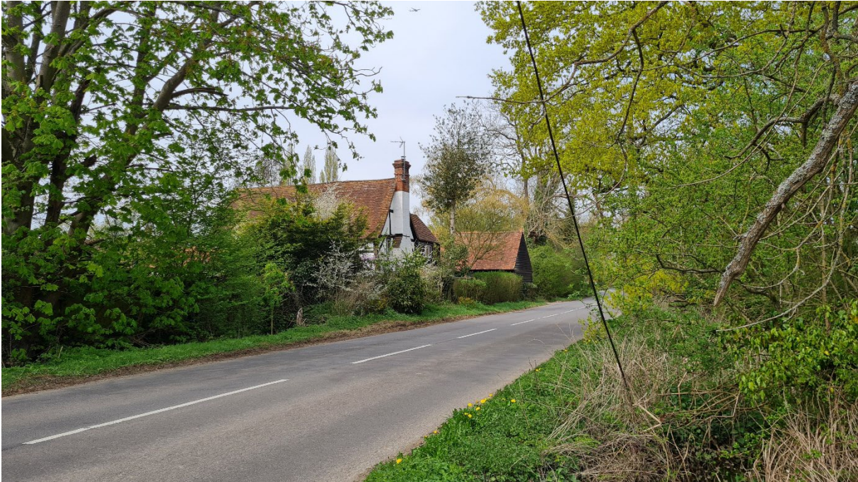
Image EDP A1.7: View of the Grade II listed Heriot ( 1117415 ) from the eastern side of the A321 road, facing north.
