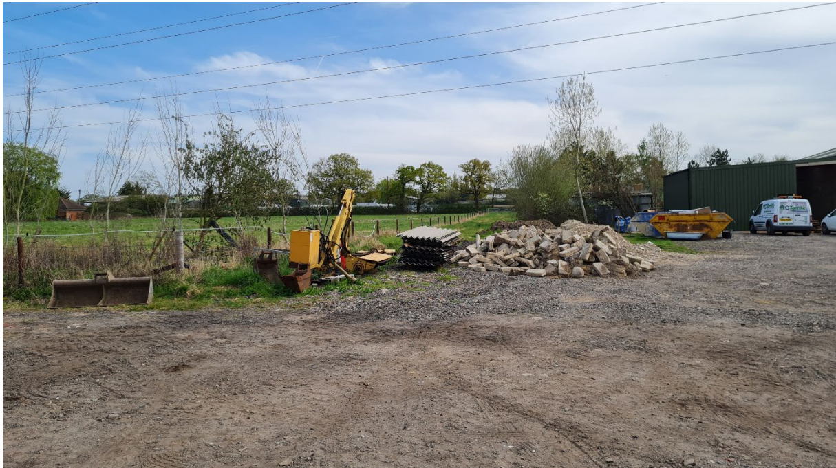
Image EDP A1.3: The site facing south-east from the yard of the commercial estate adjacent. This image shows the approximate location of one of the proposed LTM. In the background some residential and commercial units are visible, which are located along Nelson's Lane to the north. Some posts and high voltage cables are visible in the background.
