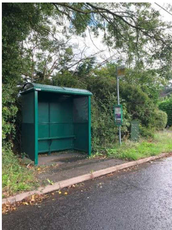
Photograph 4: Reading Road Bus Stop (eastbound)
