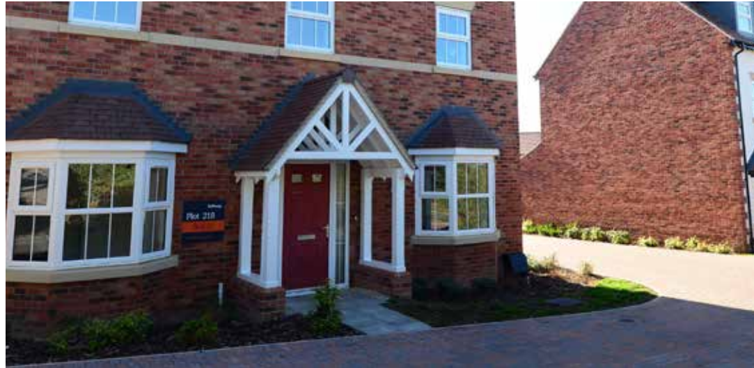
Natural coloured paving slabs to front doors.
