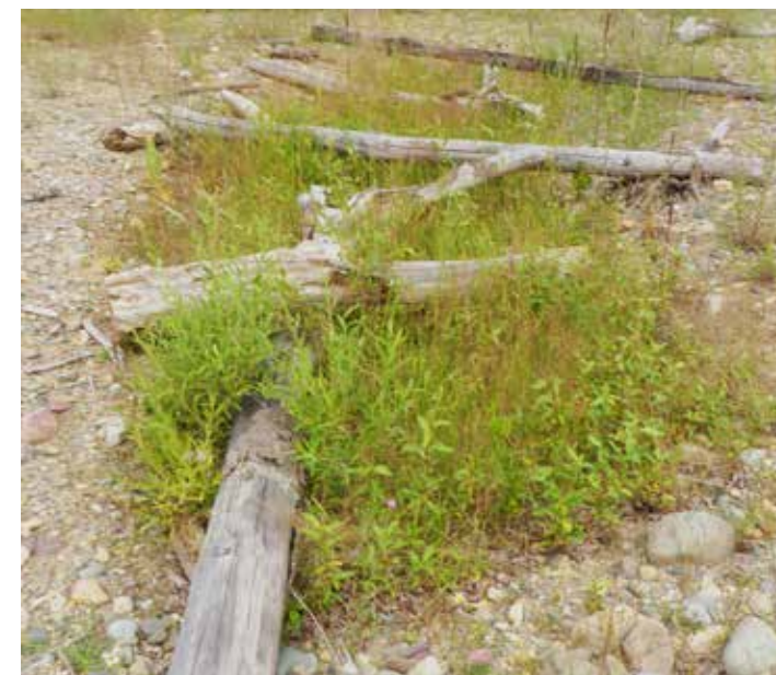
Example of timber stepping logs crossing a semi-dry SuDS feature.
