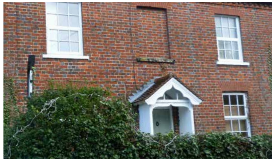
Blind window detail and central porch
