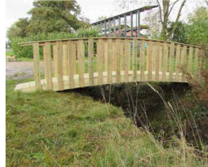
Example of a timber bridge over a ditch swale.
