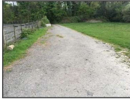
Photo 31 Compressed concrete path
