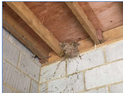
Photo 50 Bird nest inside barn (B3)
