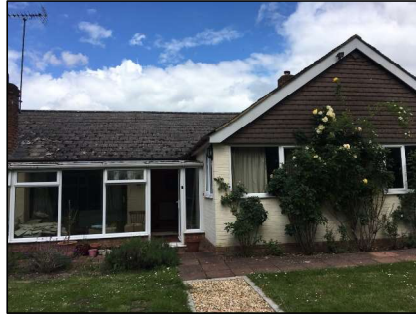
Photo 34 Residential dwelling (B1)
