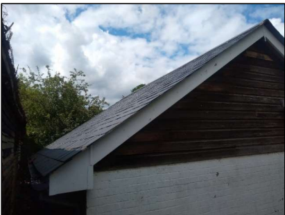
Photo 41 Brick outbuilding (B2)
