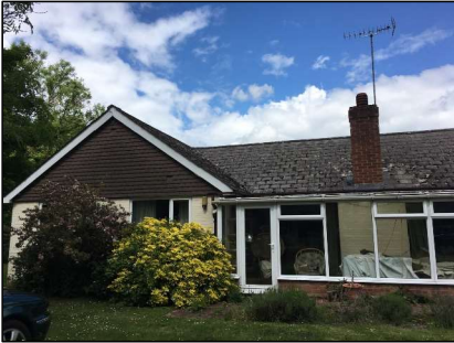
Photo 39 Residential dwelling (B1)
