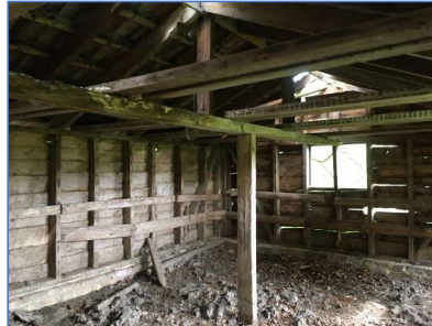
Photo 64 Timber outbuilding internals (B7)
