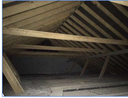
Photo 52 Barn loft void (B3)
