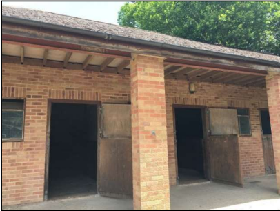
Photo 45 Barn structure (B3)
