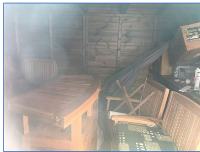
Photo 62 Timber shed internals (B6)
