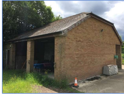
Photo 46 Barn structure (B3)
