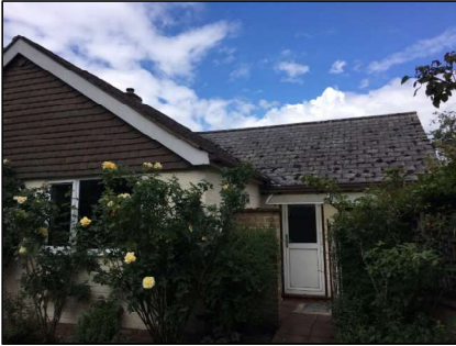
Photo 33 Residential dwelling (B1)
