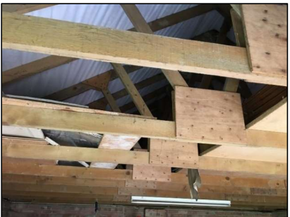
Photo 43 Internals of outbuilding (B2)
