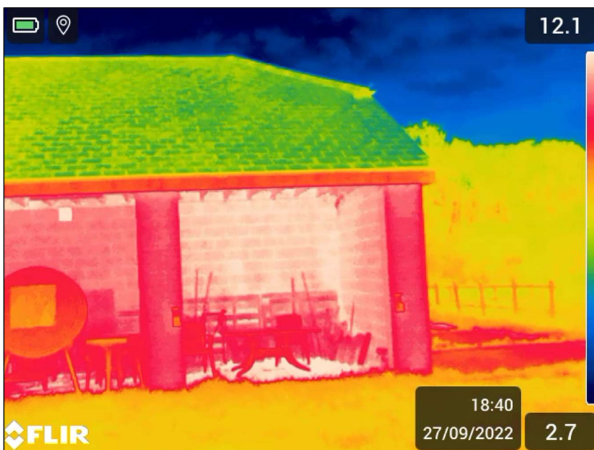
Photo 1 Eastern elevation (B3)
