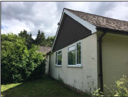
Photo 35 Residential dwelling (B1)
