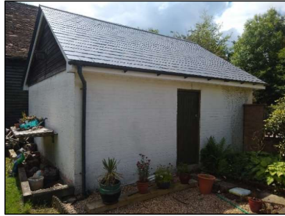
Photo 40 Brick outbuilding (B2)
