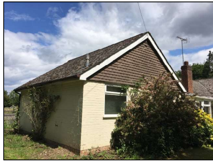
Photo 36 Residential dwelling (B1)
