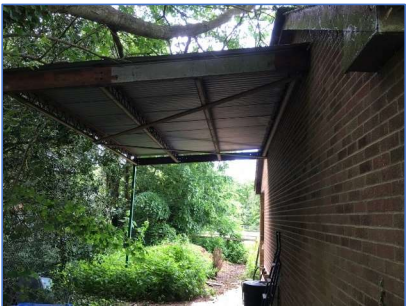
Photo 47 Barn structure (B3)
