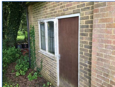
Photo 48 Barn structure (B3)
