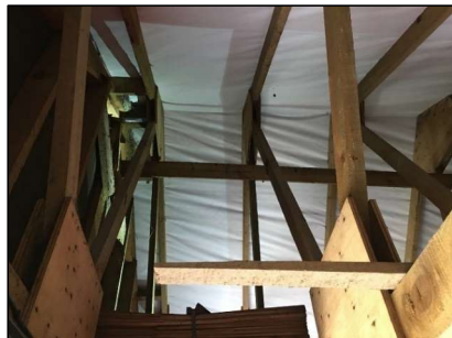
Photo 44 Internals of outbuilding (B2)
