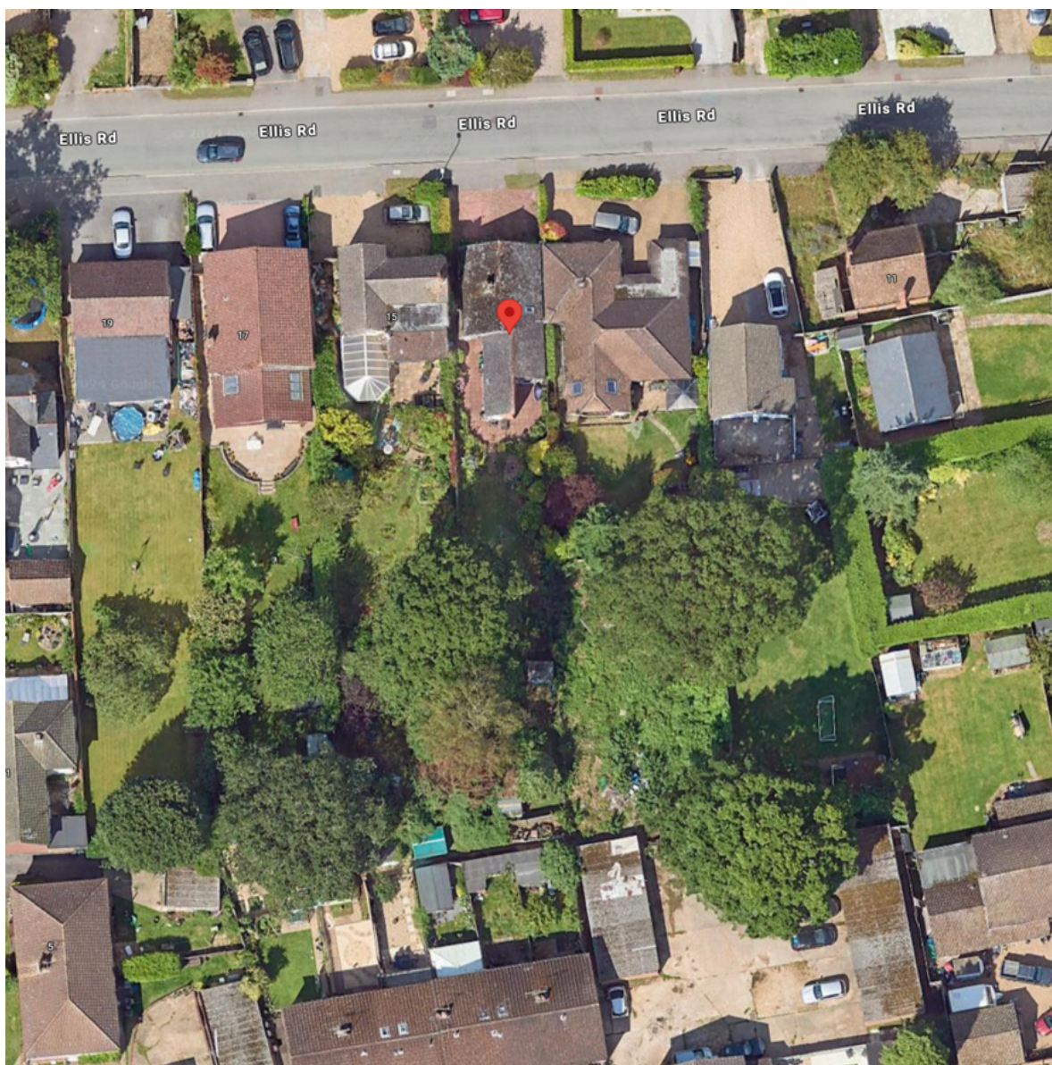
Aerial View of the proposed site
