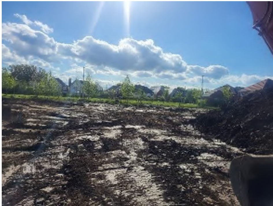
Plate 19 – Phase 3 excavation works
