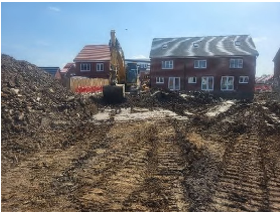
Plate 24 – Haul road removal
