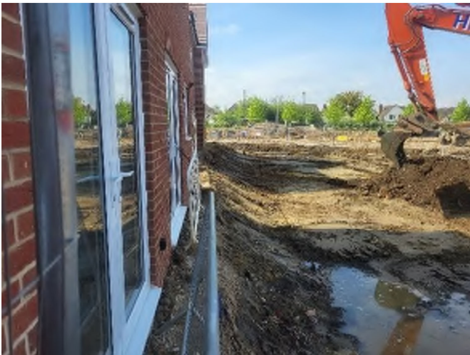
Plate 22 – Excavation of private gardens to 1mbgl, 0.5m off brickwork with 2:1 batter
