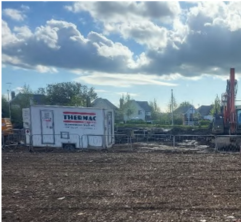
Plate 17 – Asbestos decontamination unit within segregation zone
