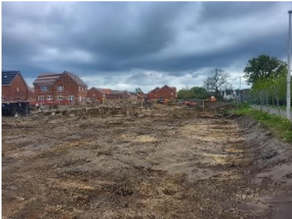
Plate 20 – Phase 3 excavation works
