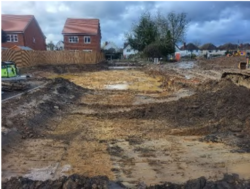
Plate 5 – Phase 1 excavation works
