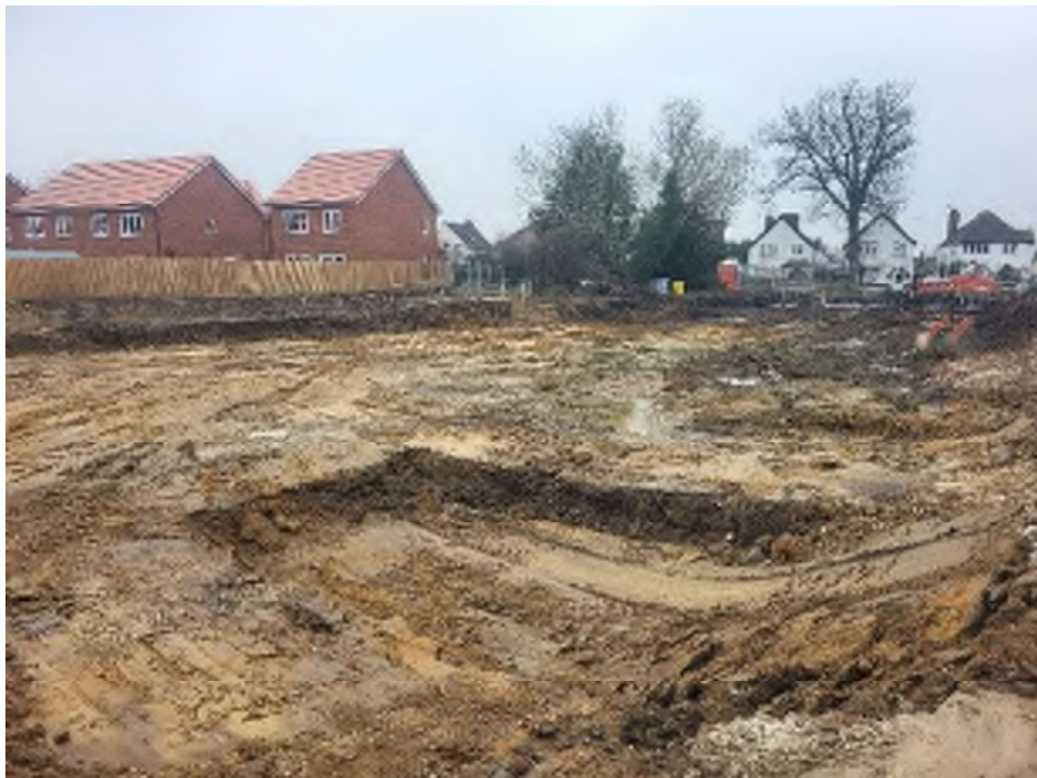
Plate 6 – Phase 1 excavation works
