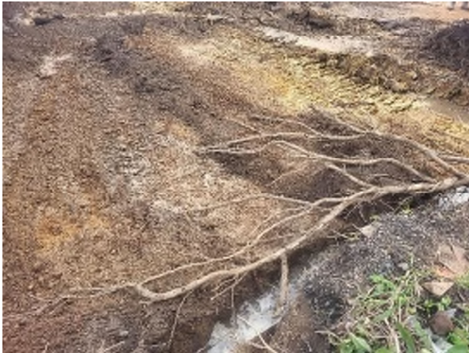
Plate 13 – TPO works, hand digging around tree roots
