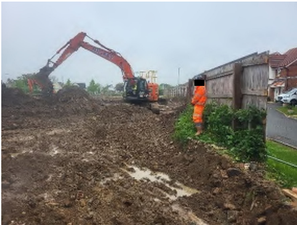
Plate 23 – Phase 4 excavation works
