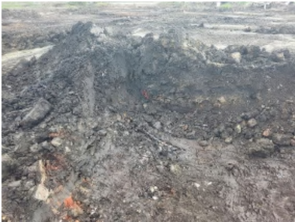
Plate 7 – Service strike during excavation
