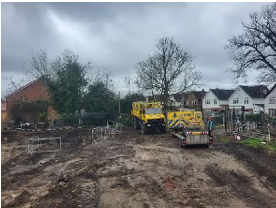
Plate 8 – Arborfield Tree Care Ltd on site to fell trees
