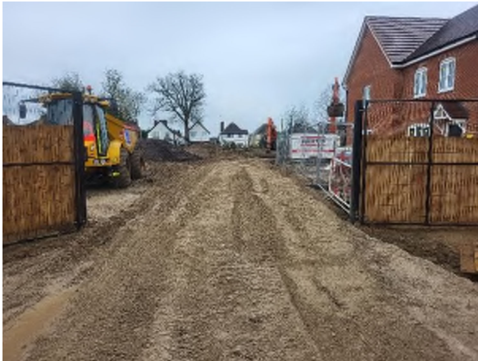
Plate 3 – Imported recycled Type 1 for haul road
