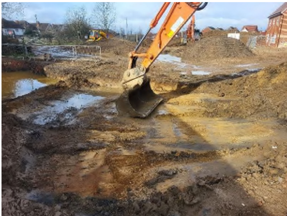
Plate 4 – Phase 1 excavation works
