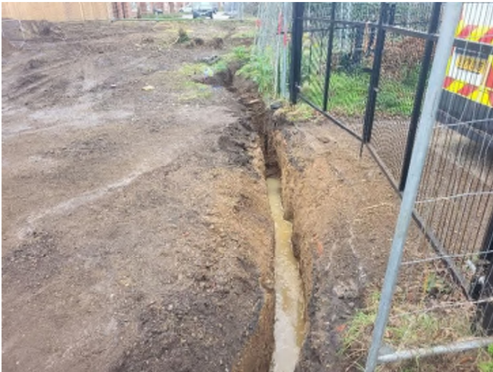
Plate 10 – Completed vacuum trench excavation
