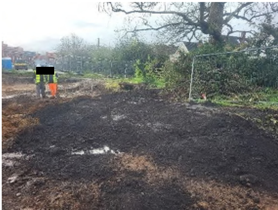
Plate 14 – Completed TPO works, backfilled with topsoil
