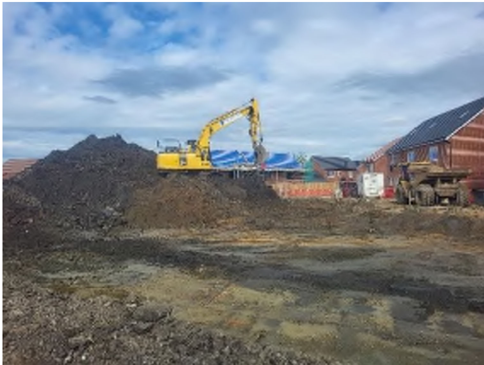
Plate 15 – Phase 2/4 excavation works
