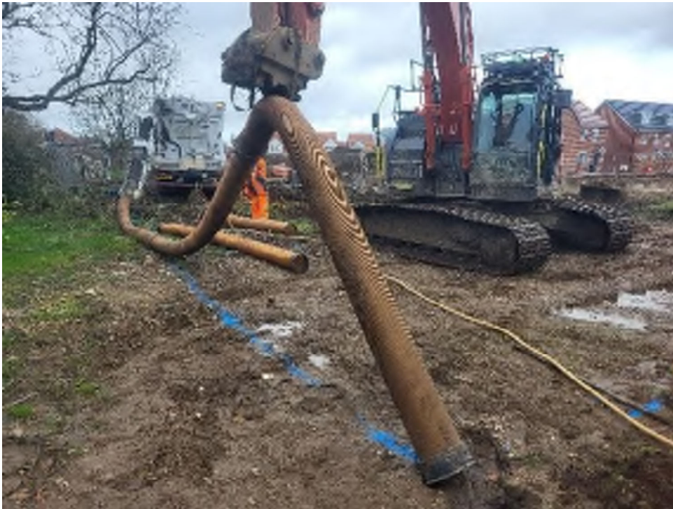
Plate 9 – Vacuum excavation of trench investigation works
