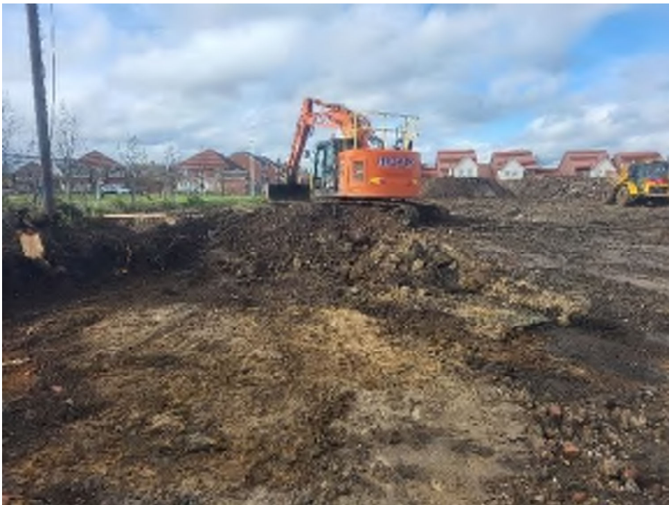
Plate 12 – Phase 2 excavation works
