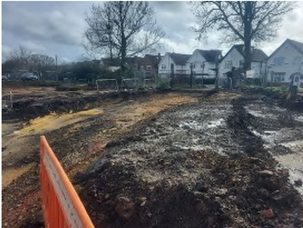
Plate 11 – Phase 2 excavation works
