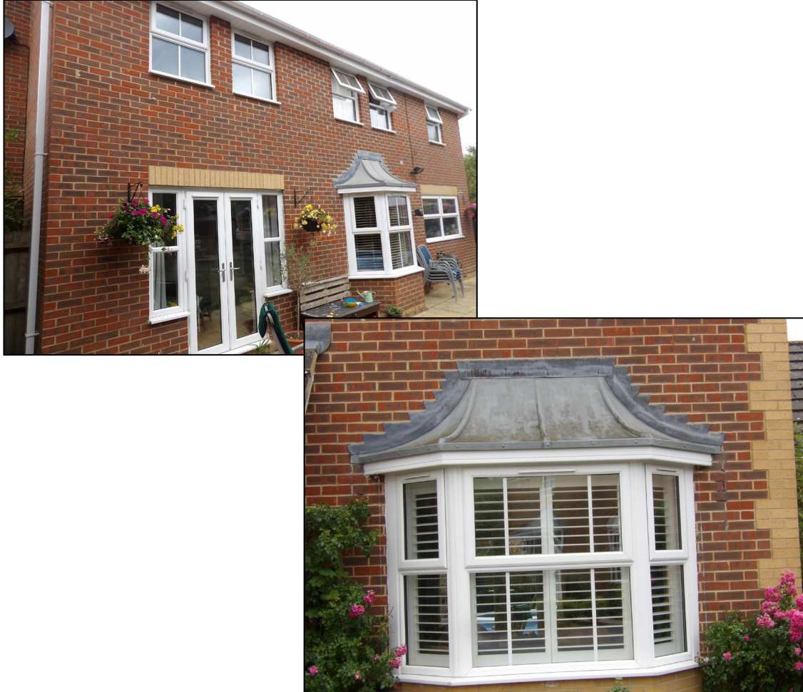
Figure 7. Rear view of property and flush lead flashing over rear, bay window. 190 Hurricane Way, Woodley. 19.08.25
