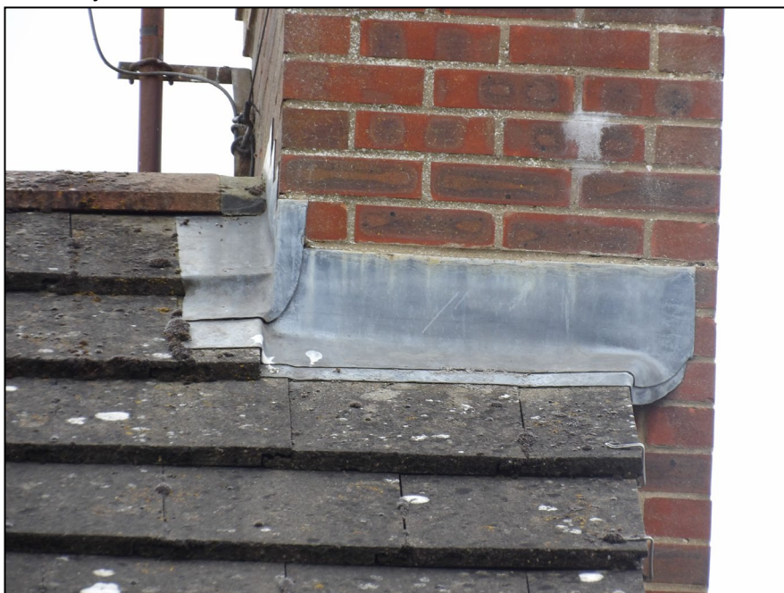
Figure 8. Example sealed lead flashing around chimney stack. 190 Hurricane Way, Woodley. 19.08.25
