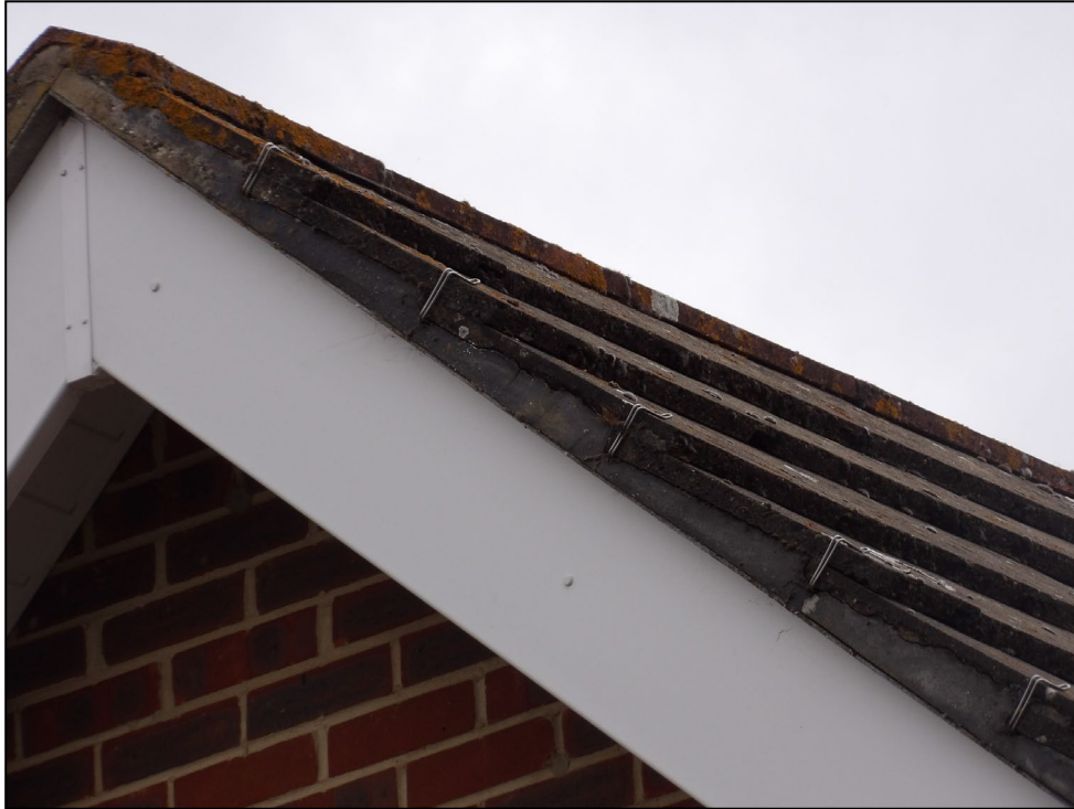
Figure 5. Example sealed verges. 190 Hurricane Way, Woodley. 19.08.25
