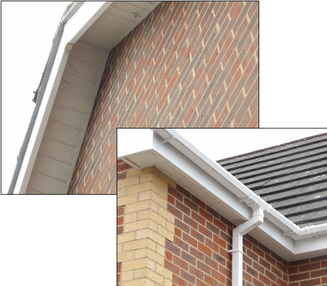
Figure 6. Example sealed uPVC soffits/fascias. 190 Hurricane Way, Woodley. 19.08.25
