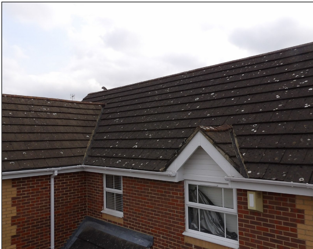
Figure 4. Example of roof and ridge tiles. 190 Hurricane Way, Woodley. 19.08.25
