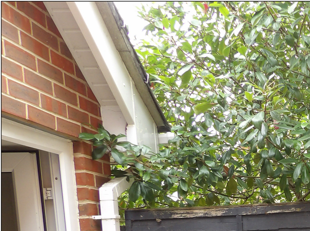
Figure 10. Example sealed soffits/fascias/verges on garage. 190 Hurricane Way, Woodley. 19.08.25
