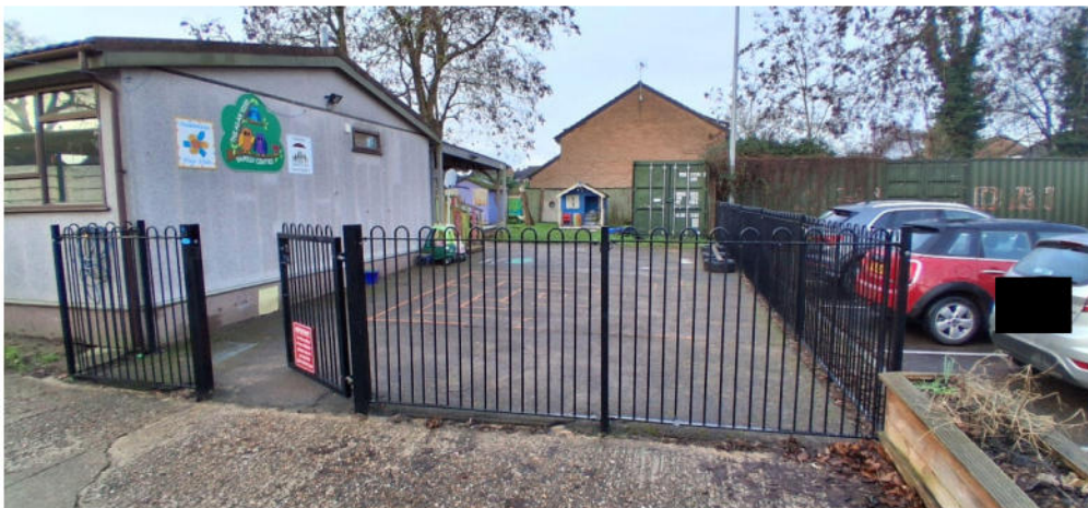
Existing nursery and hard surfaced play area
