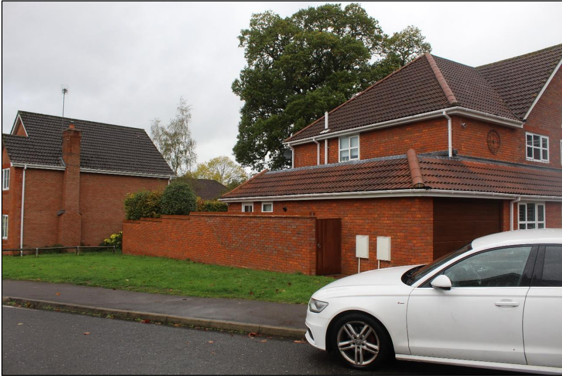
Photograph 2 – Side elevation as viewed from Twycross Road
