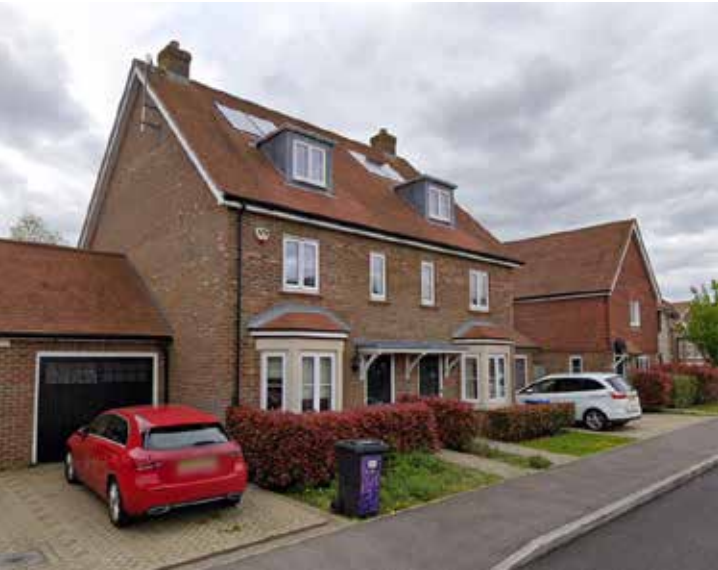
Form of the dormer windows with flat roofs
