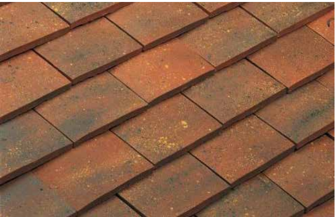
Roof - Orange Clay Tile
