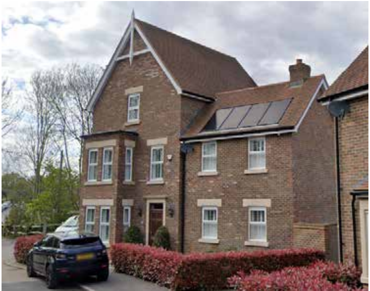
Overall building mass with the gable fronted 3 storey section and false chimney to the 2 storey section
