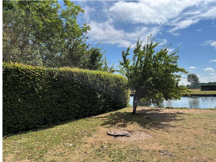
Figure 3: Location of Existing Foul Sewage Tank (under the manhole seen in photo above)
