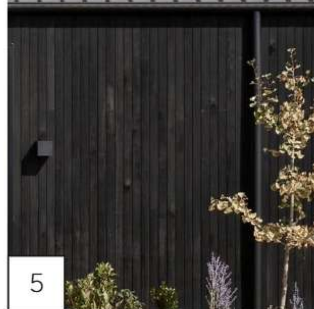
Charred Timber Cladding
