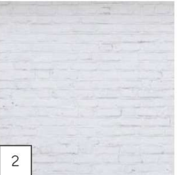
Painted White Brickwork
