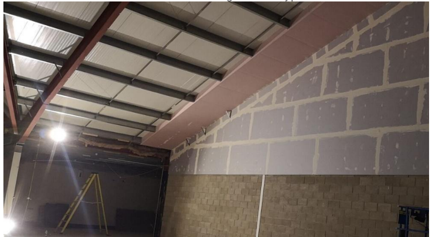
Figure A – Typical Acoustic Bulkhead
