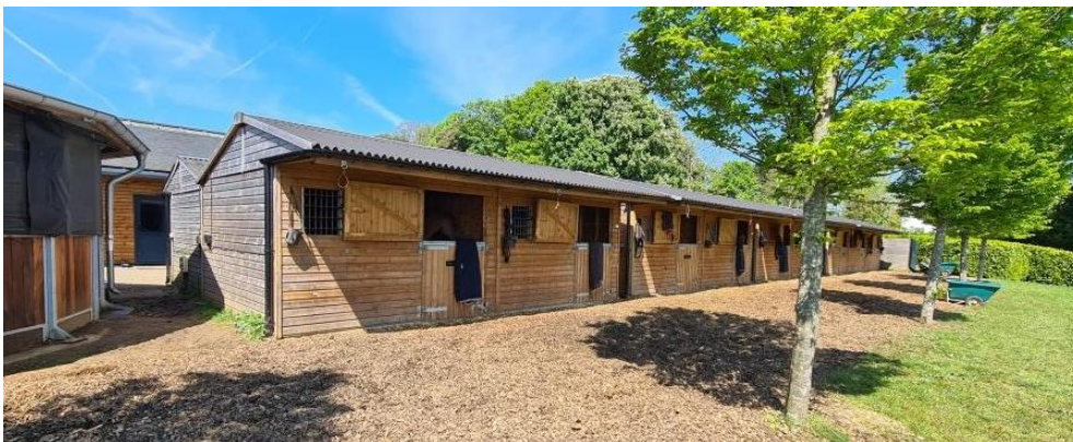
Fig. 11 – The row of looseboxes (Block C)
