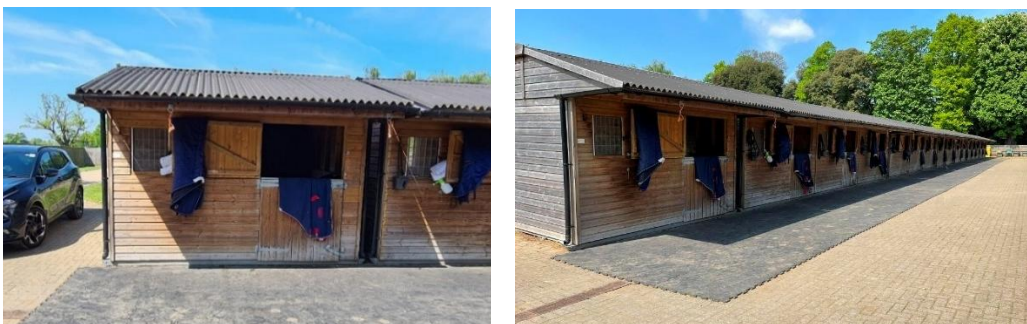
Fig. 12 – The single loosebox unit (situated on the end of existing row of stable Block A)
