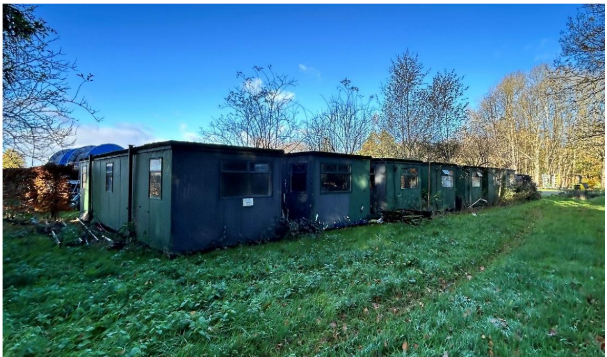
Fig. 3 – The portacabin buildings proposed to be traded-off (rear elevation)
